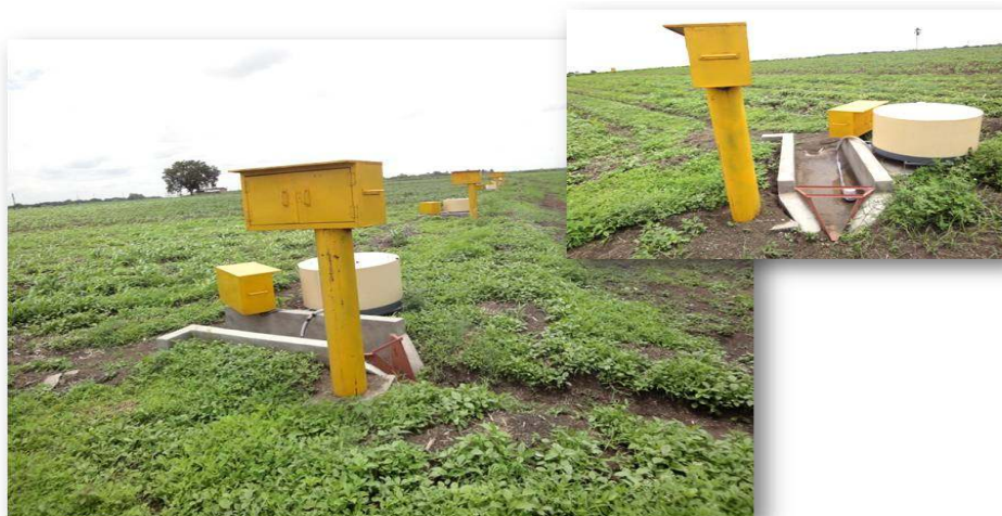
Fig. 2. A field view of the installed integrated digital runoff and soil loss monitoring unit (IDRSMU), photo in insert is close up of IDRSMU
