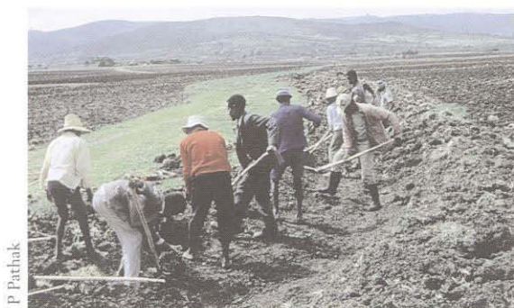
Farmers build the main drainage channel at Ginchi.
