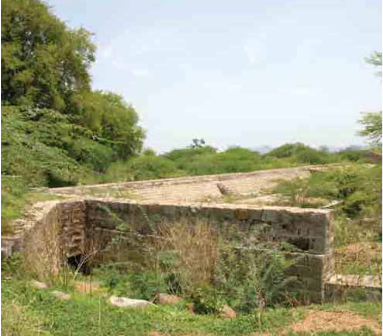
A check dam built under the watershed management program.
