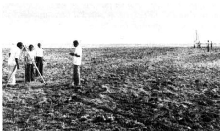
Figure 3. A detailed topographic survey is a prerequisite for planning land development, to decide upon roads and field drains and to execute land smoothing.
