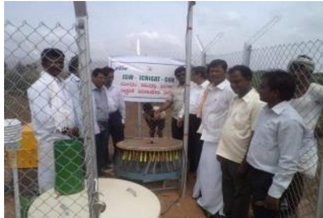
Figure 49. Installation of Hydrological gauging station at JSW villages
