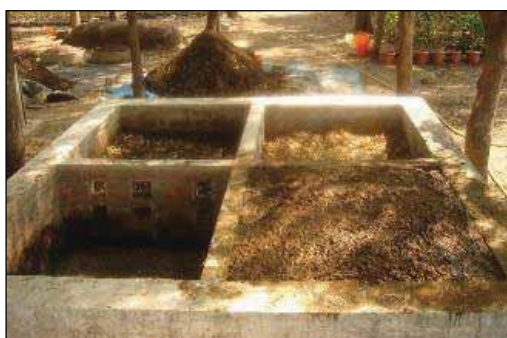
Fig. 5. ICRISAT commercial model with four chambers showing different stages of vermicomposting (left) and diagram showing the cycle of composting and movement of earth worms (right) Source: Nagavallema et al. (2004).
