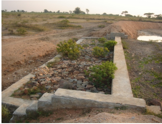
Figure 3. PT filled with sediment (left) and CD developed leakages (right), Pragathi watershed
