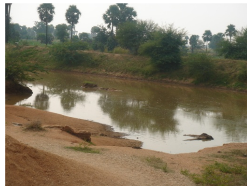
Fig Check dam and Percolation tank improved ground water level of wells and bore wells of farmers around the area but not so effective needs removal of silt clearing bushes around.
