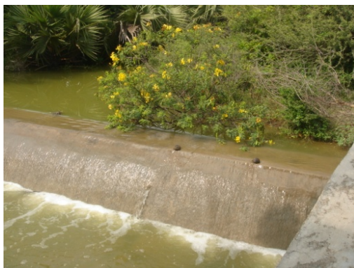
Fig Check dam and Percolation tank improved ground water level of wells and bore wells of farmers around the area but not so effective needs removal of silt clearing bushes around.
