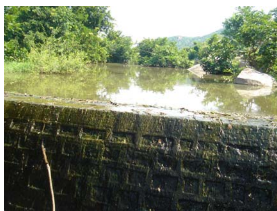
Fig: Check dam constructed near Srinivasreddy field
