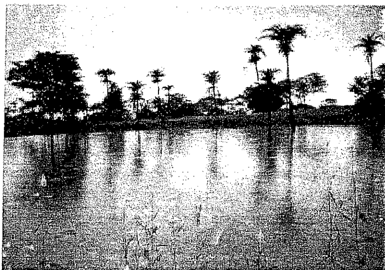
Fig. 5. An earthen check dam at Lalatora watershed, Madhya Pradesh, India
