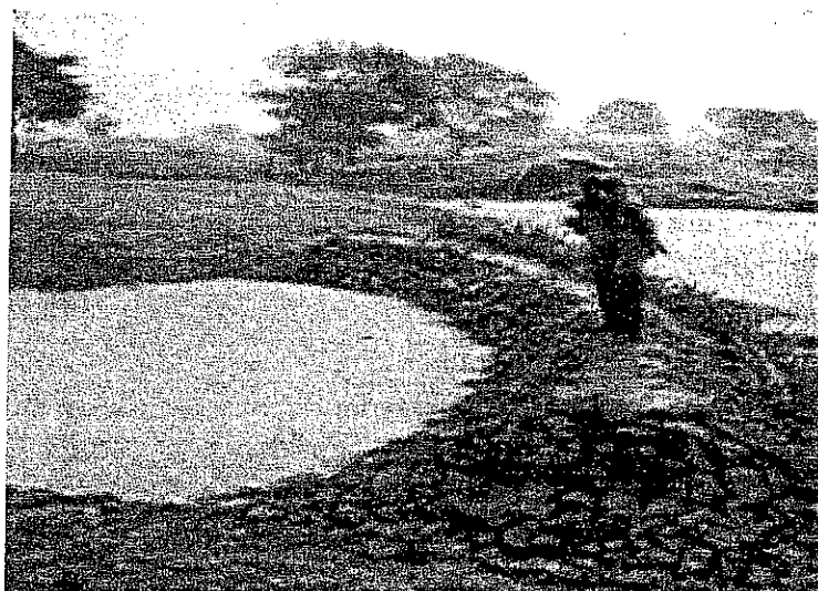
Fig. 6. A low-cost mini percolation tank (earthen structure) at Adarsha watershed, Kothapally, Andhra Pradesh
