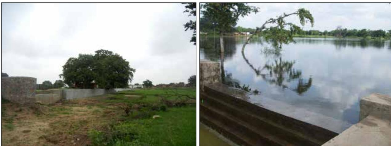
Figure 2. Haveli renovation in Parasai-Sindh watershed; Masonry drop spillway (rectangular weir) and embankment along with core wall was constructed in 50 m breached area. Water harvested in Haveli during the monsoon period.
