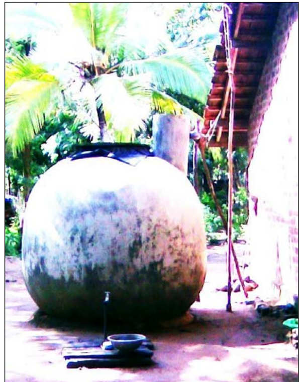
Figure 7. Water harvesting tank in a house at Galahitiyagama.
