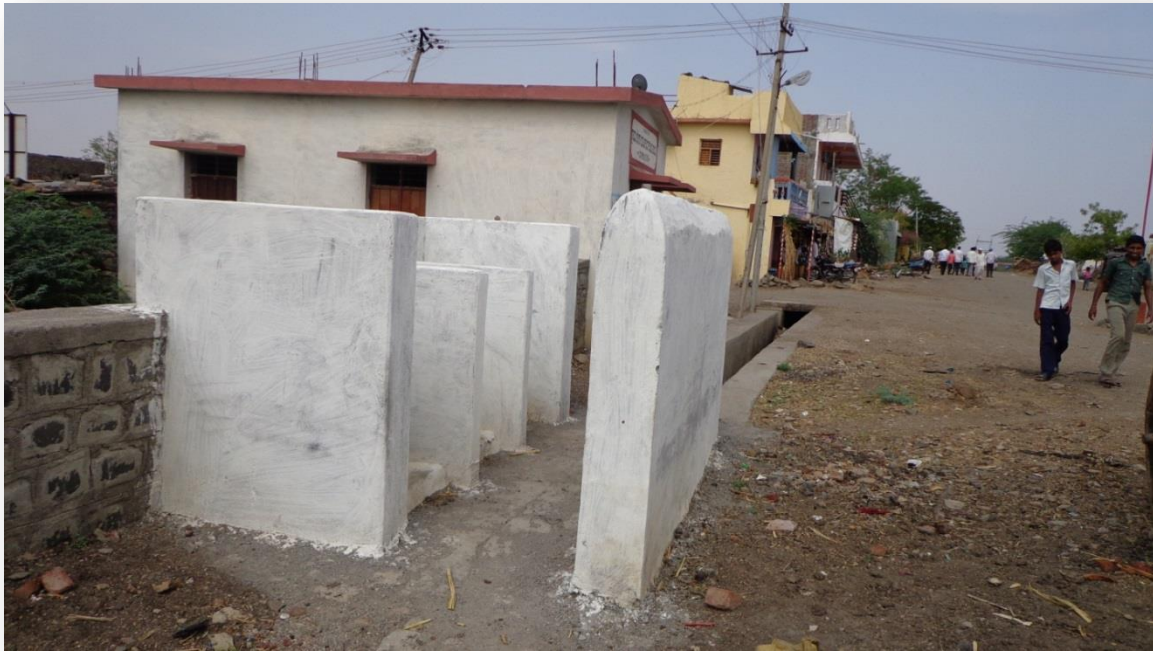
Plate 3: Public toilet constructed under MGNREGP in Markabbinahalli village. [Dated 10-05-2013]
