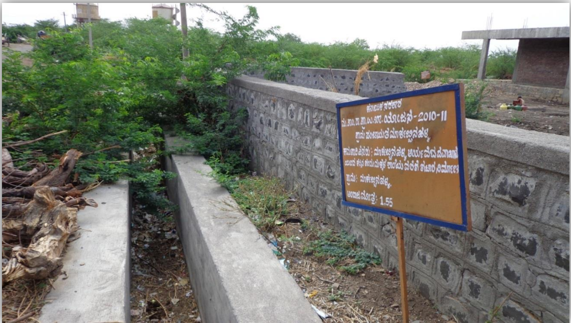
Plate 2: Drainage constructed under MGNREGP in Markabbinahalli village. [Dated 10-05-2013]
