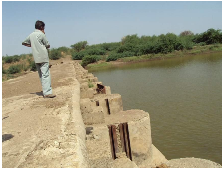
Check dam and canals in 1990's opened the way for surface water use to climate proof agriculture in Shirapur village, Maharashtra, India
