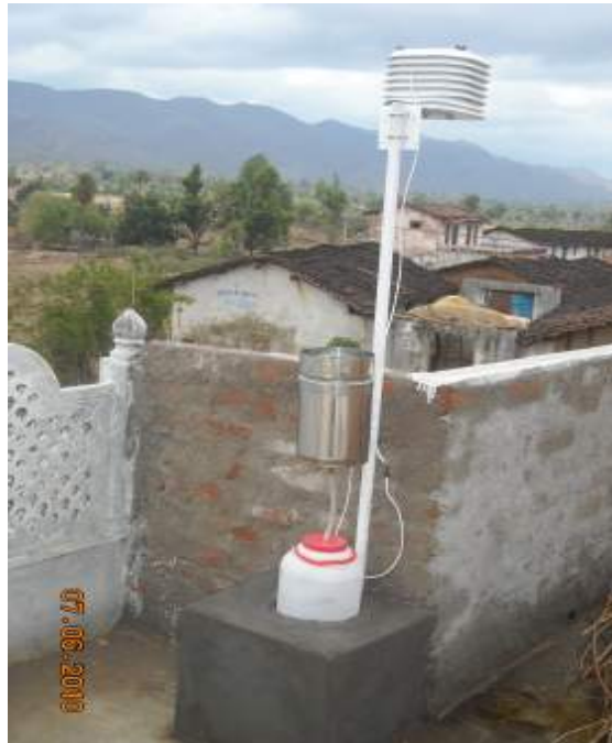
Figure 6. Rain gauge installed at the Dob-Navaj model watershed, Udaipur district
