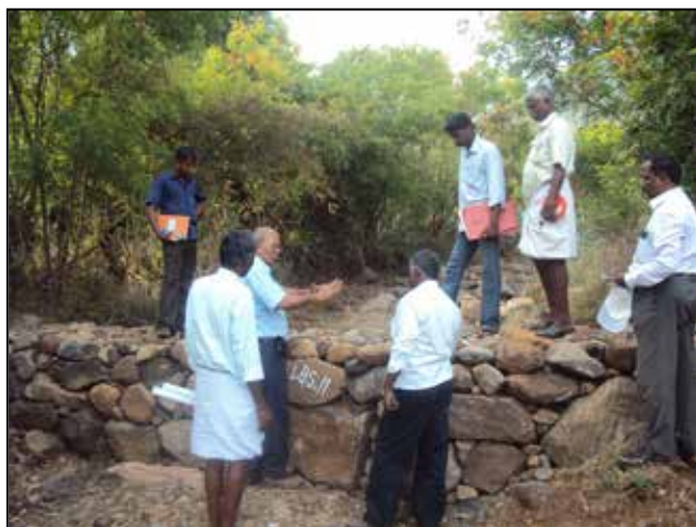
Loose boulder structure
