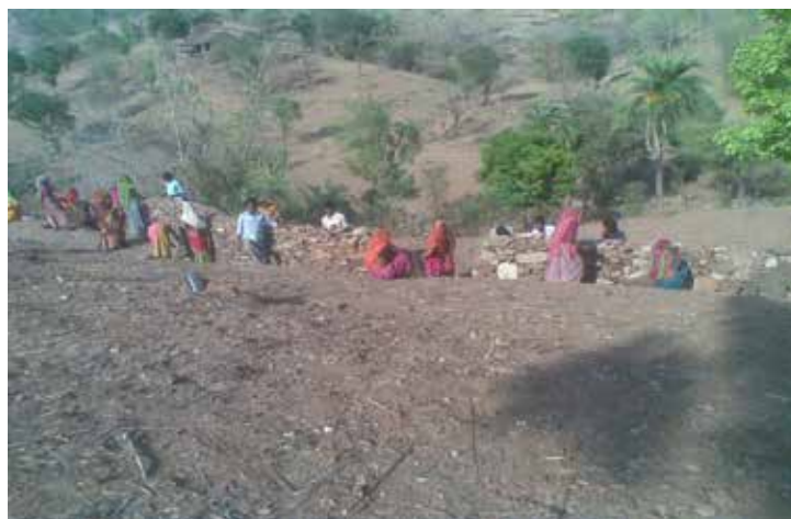
Figure 16. Construction of Joint forest management boundary wall work in Nevaj village
