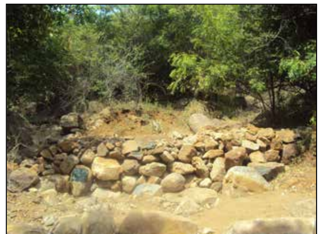
Loose stone structure
