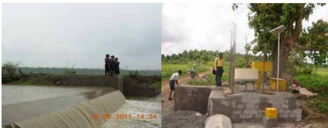
Figure 9. Runoff and soil loss measuring structure and equipments at Padarlya-Siyalwada model watershed, Raisen district.
