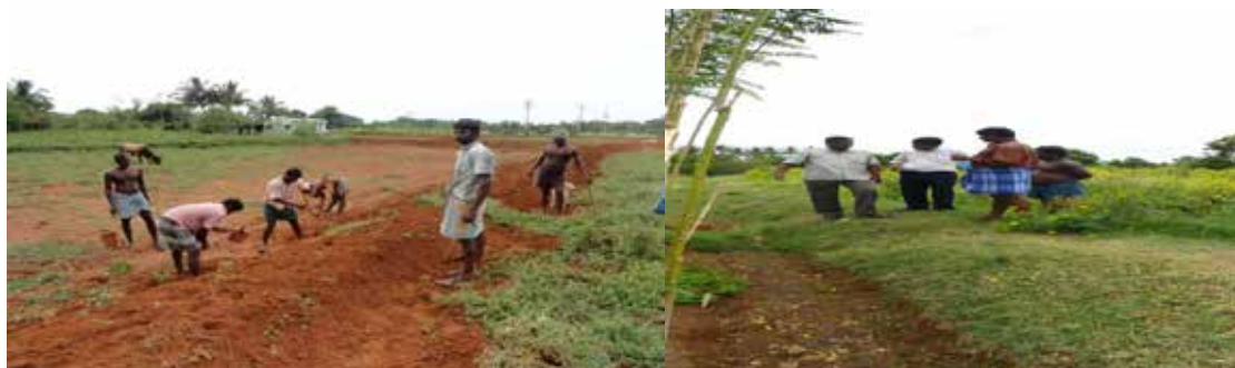
Figure 24d. Field bunding
