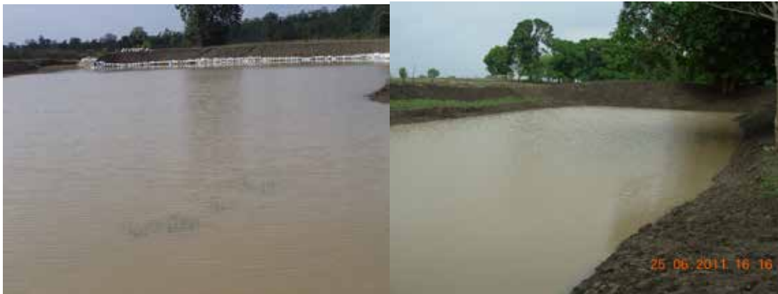
Figure 10. construction of ponds and earthen check dams at Siyalwada village, Raisen model watershed.
