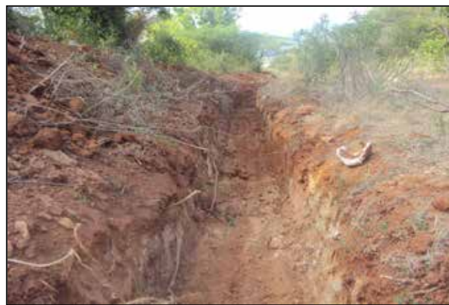
Figure 27. Diversion drain below foot hills of forest to divert runoff from Sirumalai forest
