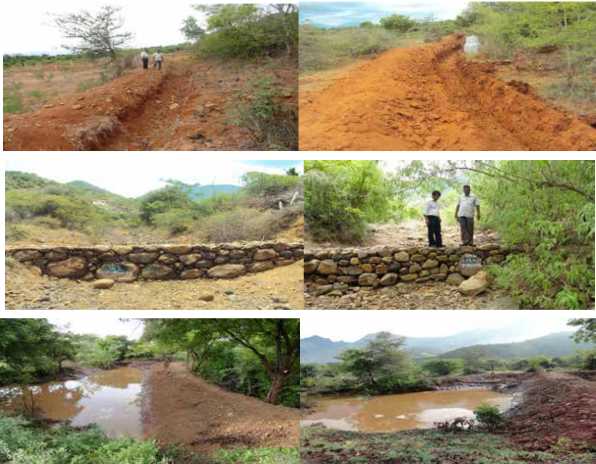
Figure 24a. Gully control structures constructed at model watershed
