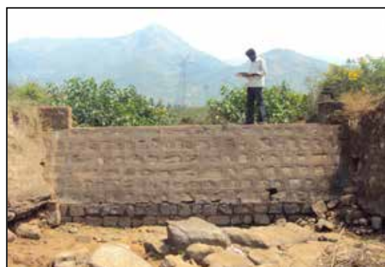
Figure 10. Existing weir structure in the watershed
