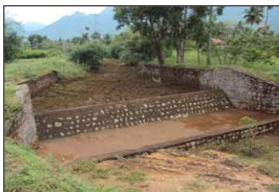
Figure 9. An existing masonry check dam in the watershed
