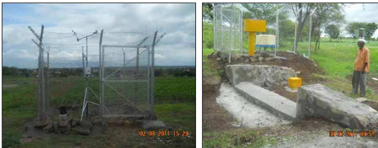
Figure 12. Automatic weather and Hydrological gauging station with micro processor based integrated runoff recorder and sediment sampling unit installed at Dolasne-Bambalwadi Model watershed.
