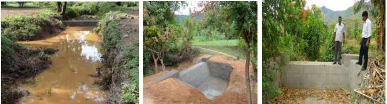
Figure 24b. Masonry check dams
