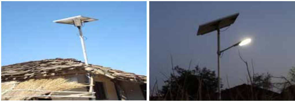
Figure 18. Solar powered street lights in Dungaria village of model watershed, Raisen District, Madhya Pradesh
