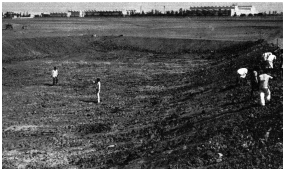
Figure 99. Final shaping of side slopes of the tank and tank bund.
