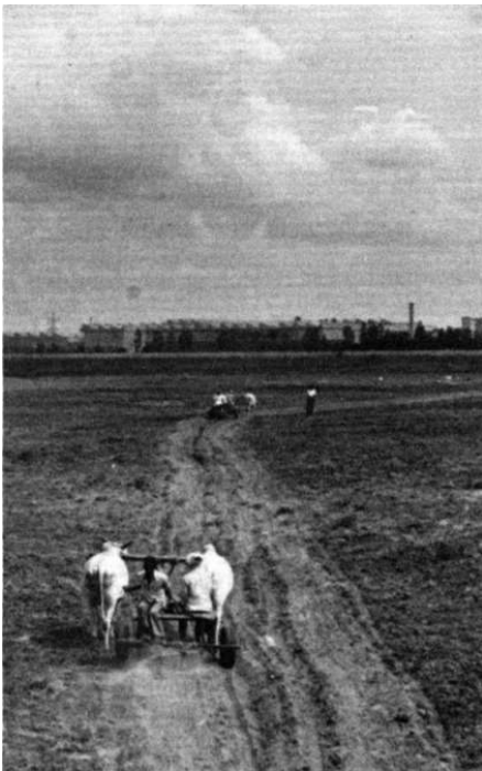
Figure 97. Wheeled tool carrier fitted with angle blade is used to construct a grassed waterway on an Alfisol watershed.
