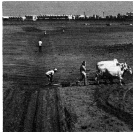
Figure 98. An indigenous wooden scraper is used for final shaping of the grassed waterway and deposition of excess soil in microrelief depressions.
