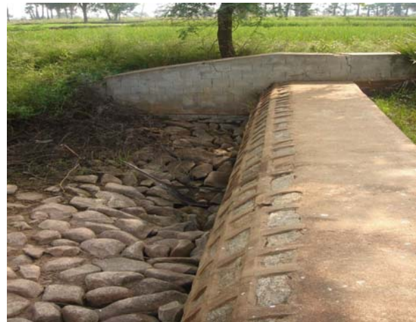
Figure 2. A big hole on wing wall (left) and damage on apron wall (right) of check dams, Kandikunta watershed, N G Kothapally village, Shaligouraram Mandal
