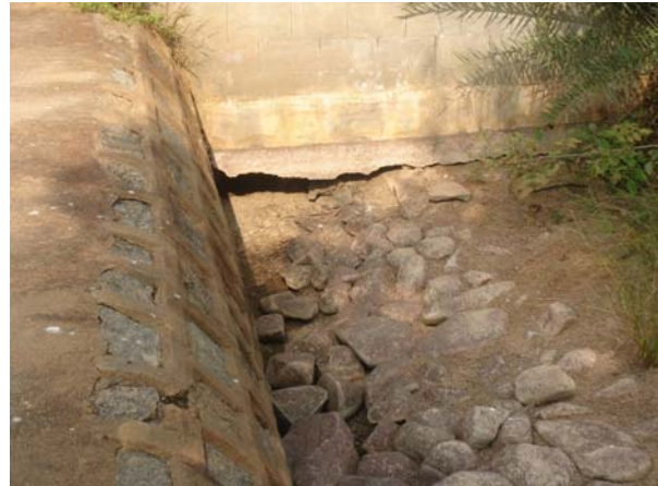
Figure 2. Damages on wing wall and apron wall of check dam, Gorekunta watershed, N G Kothapally village, Shaligouraram Mandal
