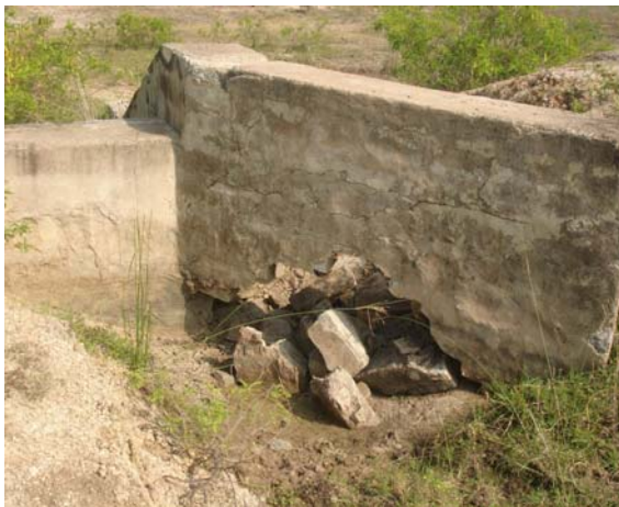
Figure 2. A big hole on wing wall (left) and damage on apron wall (right) of check dams, Kandikunta watershed, N G Kothapally village, Shaligouraram Mandal
