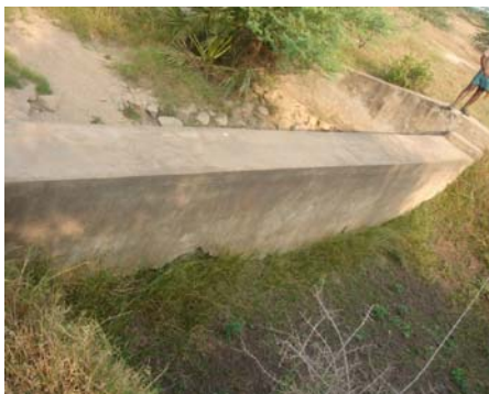
Figure 2. Damages on apron wall, leakages from check dam and grown up bushes, silt deposition in the structures at Jammikunta watershed, Shaligouraram Mandal
