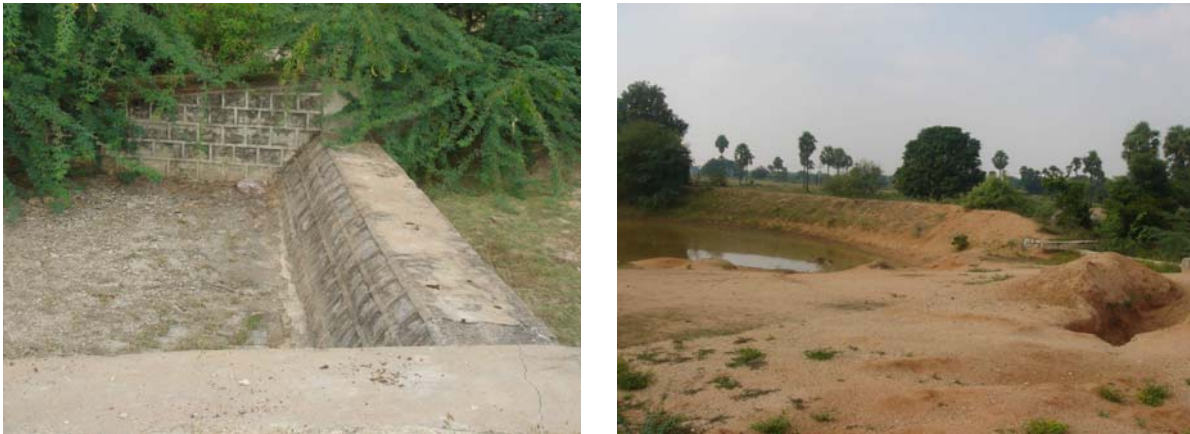
Figure 1. Check dam (left) and percolation tank (right) at Hanuman watershed, Mothey Mandal.
