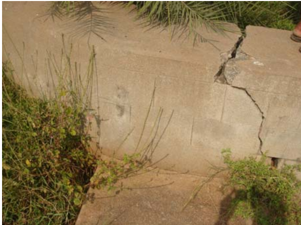
Figure 2. Damages on wing wall and apron wall of check dam, Gorekunta watershed, N G Kothapally village, Shaligouraram Mandal
