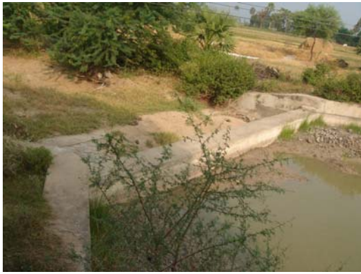
Figure 1. Masonry check dam (left) and damaged percolation tank (right) at Kisan watershed, Adloor village, Shaligouraram Mandal.
