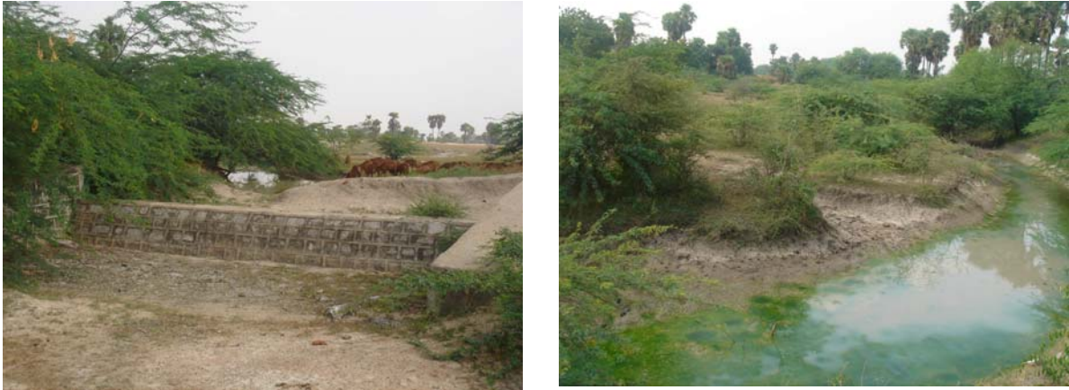
Figure 1. Check dam (left) and percolation tank (right) at Bairavudu watershed, Shaligouraram Mandal.
