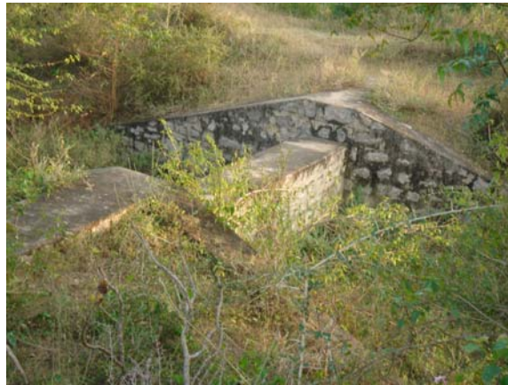
Figure 2. Masonry check filled with bushes at Gummadavalli watershed, Thungathuthy Mandal
