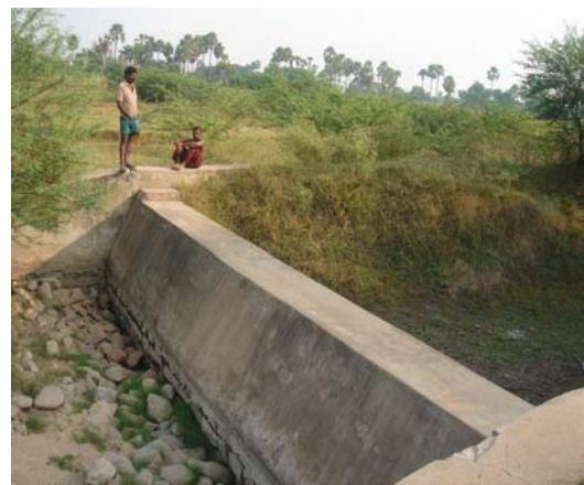
Figure 2. Damages on apron walls and leakages from check dams, Kisan watershed, Adloor village, Shaligouraram Mandal
