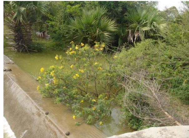
Figure 2. Damage on apron wall and encroachment of bushes in check dams, Voorakunta watershed
