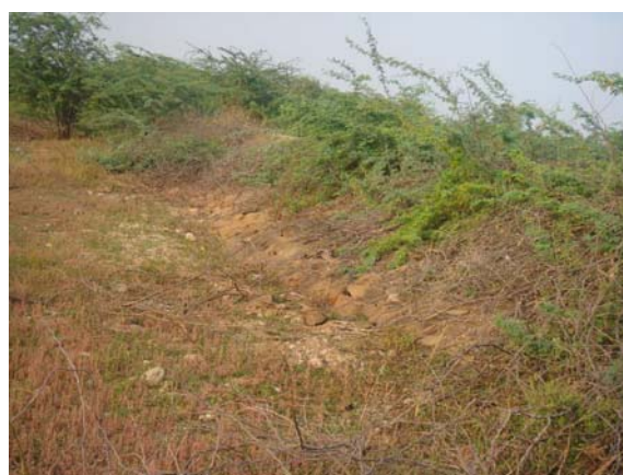
Figure 2. Percolation tank with stone revetment at Karshak watershed, Akaram village, Shaligouraram Mandal
