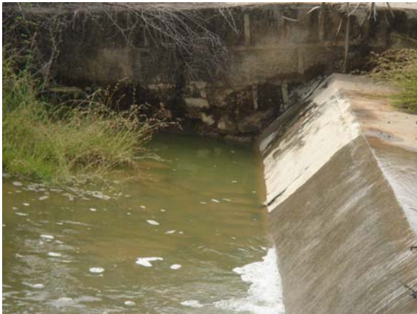
Figure 2. Damage on apron wall and encroachment of bushes in check dams, Voorakunta watershed
