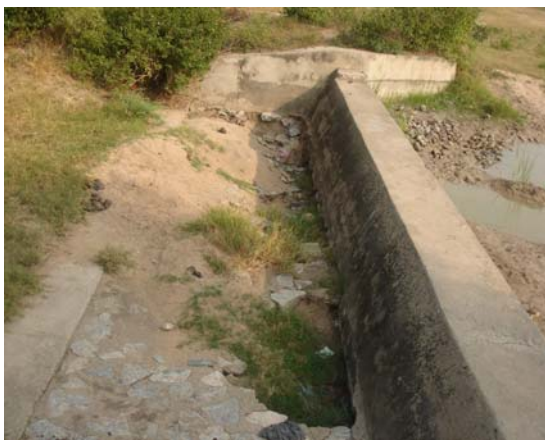
Figure 2. Damages on apron walls and leakages from check dams, Kisan watershed, Adloor village, Shaligouraram Mandal
