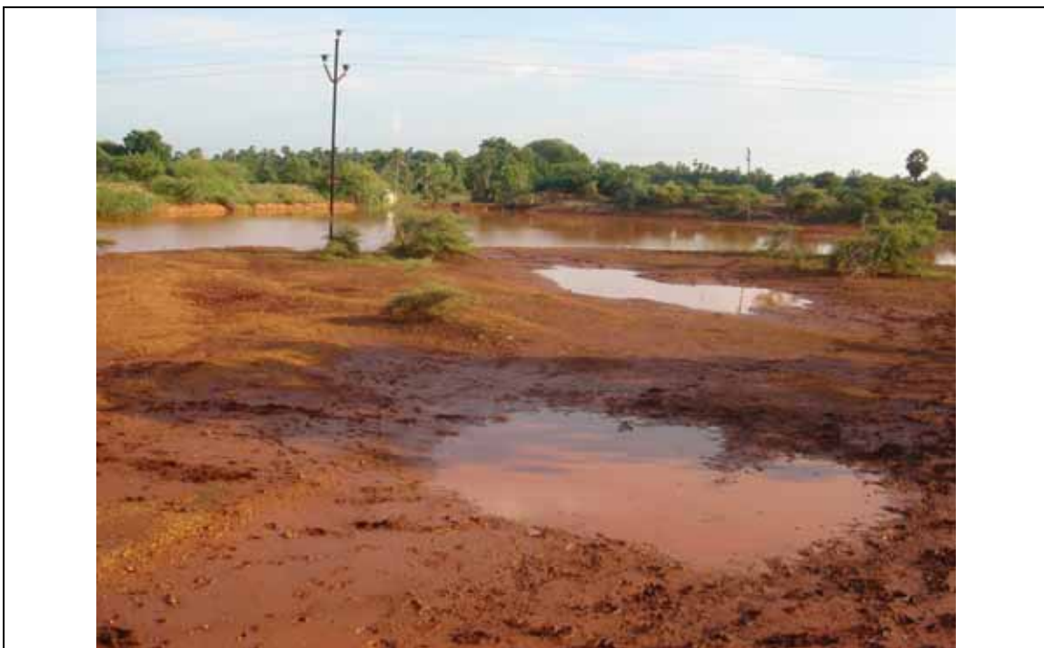
Picture 18. A percolation tank in Veerankallu developed during IWDP Phase III with approximately 60 m 3 of water during October 2009, before the start of NE monsoon rains.
