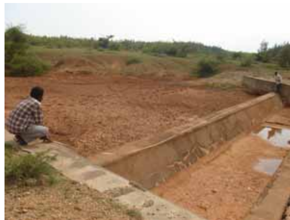
Picture 4. A big masonry check dam located on Mondikunta vagu was silted reducing storage capacity, needs desilting.
