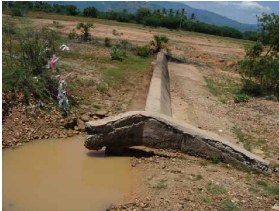
Picture 9. A masonry check dam located on Basava tank kaluju kaluva was constructed but serves no purpose as quality of structure was poor and embankment was also not properly done in Paravolu watershed, Venkatagiri Mandal, Nellore district
