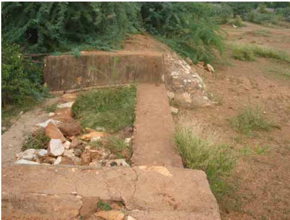
Picture 15. Masonry checkdam located on Mangalakunta vagu can be effective in conserving runoff water and recharging groundwater, 10 beneficiary farmers around the structure with 4 open wells and 3 bore wells in Tellapadu watershed, Kaligiri Mandal, Nellore.
