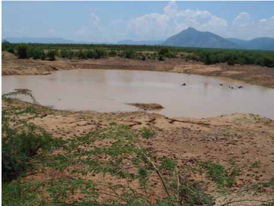
Picture 10. A percolation tank (Ramaswamy kunta) with 400 m 3 stored water was effective in conserving water and recharging groundwater. 13 bore wells are operational irrigating 48 ha of land.
