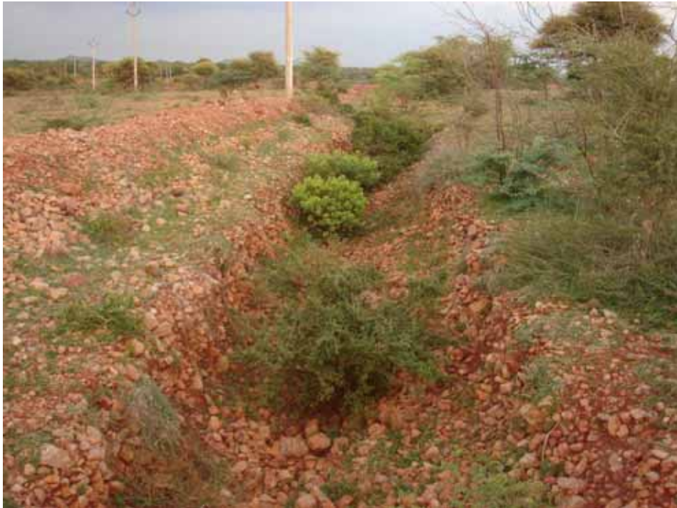
Picture 1. Continuous contour trench at the upper terrain around a hillock at Chakalikonda, Vinjamur mandal, Nellore district.
