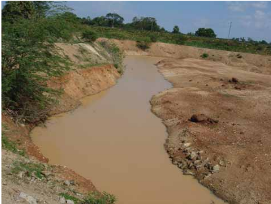
Picture 13. A percolation tank (Kotha kunta) with 800 m 3 capacity as its outlet left bare without stone pitching or any treatment.
