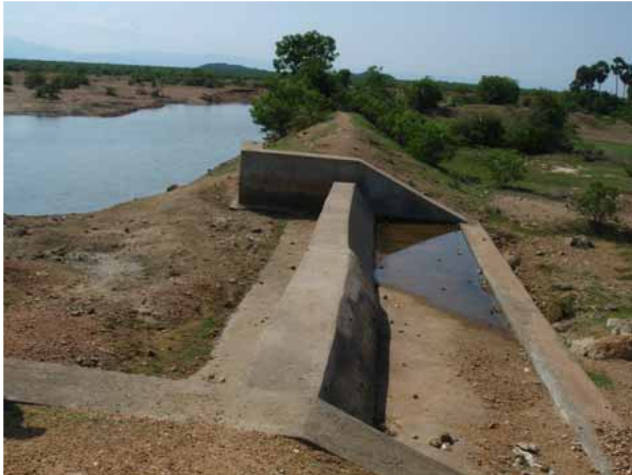
Picture 14. Percolation tank with surplus weir (on Peenugula kaluva), water stored was used for irrigating paddy fields in the down stream area.
