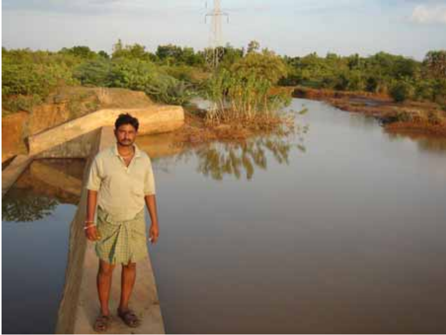
Picture 5. A masonry check dam constructed on Eduru kaluva (about 500 m 3 water storage capacity) has 200 m 3 water serves 20 open and 7 borewells in Kanuru watershed, Pellakur mandal, Nellore district.
