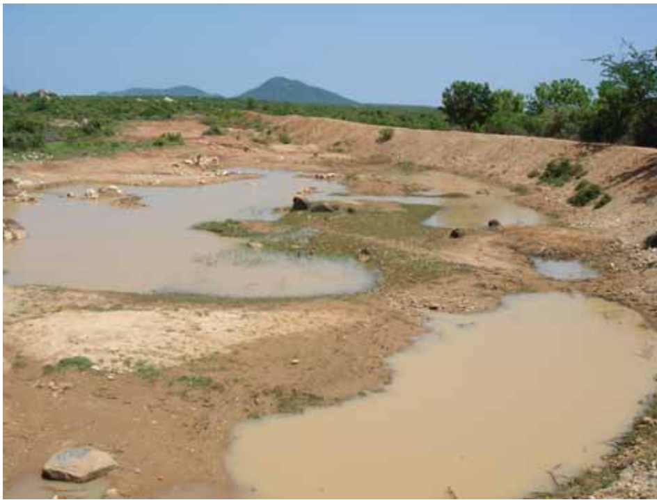
Picture 7. Percolation tank at Madigakunta has the storage capacity of 500 m 3 of water, serves 5 open wells and 20 bore wells benefiting 20 farmers in Madhavayapalem, Dakkili mandal, Nellore district..
