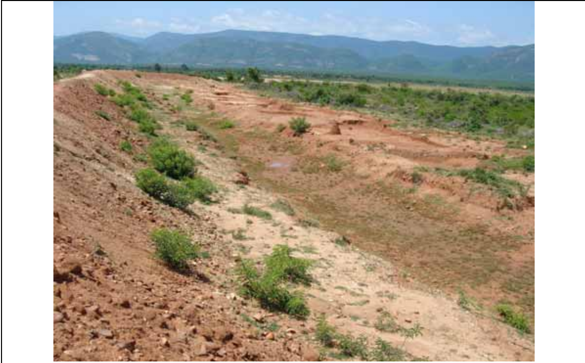
Picture 8. Percolation tank II at Jeeva Kunta has a capacity of 350 cubic meters of water, located in a catchment area of Velikondalu tank and slope is in the opposite direction to the bund and serves no beneficiaries(Madhavayapalem, Dakkili mandal, Nellore).
