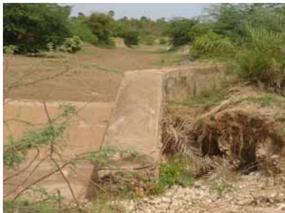
Picture 3. A check dam on Alugu vagu silt deposited and breaching at the side-wall in Chinna Annaluru watershed, Kaligiri Mandal, Nellore.
