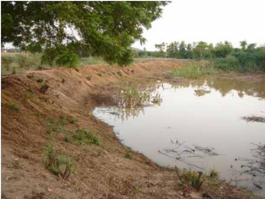
Picture 6. An old percolation tank (Bopana kunta) was renovated under IWDP III project serves 8 open wells in the surroundings in Kanuru watershed, Pellakur mandal, Nellore.
