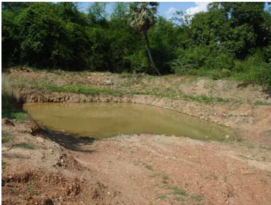
Picture 12. A mini-percolation tank (Gajulavari kunta) of about 300 m 3 , quality of construction was good in Pigilam watershed, Balayapalli mandal, Nellore district.
