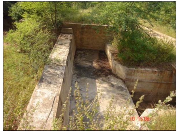
Picture 13. Masonry check dams constructed in the forest lands in Ponnala watershed.
