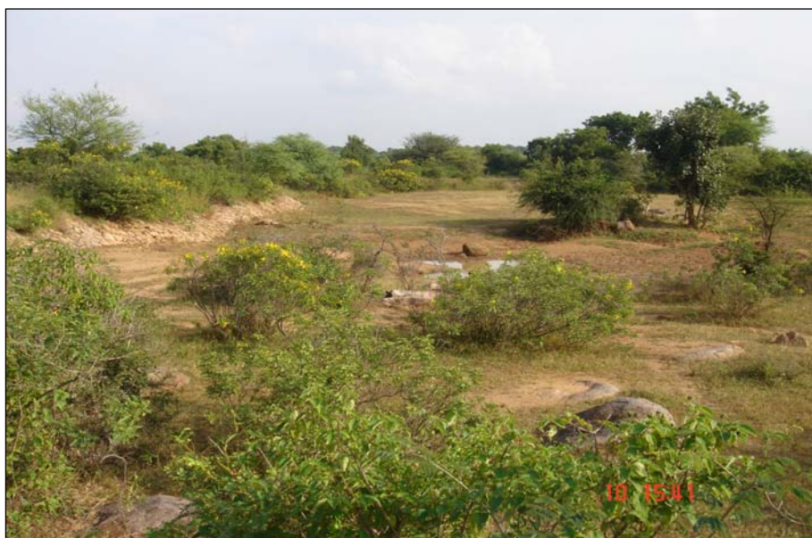
Picture 14. Percolation tank constructed in Tadkapally watershed, Medak district.
