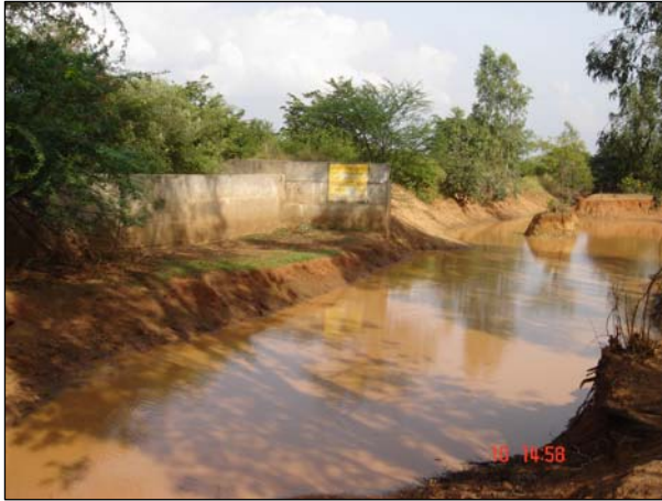
Picture 13. Masonry check dams constructed in the forest lands in Ponnala watershed.
