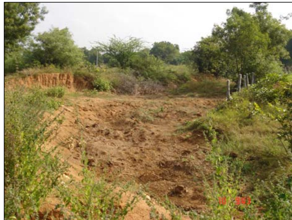
Picture 5. Filled up PT constructed on Gudikandula village cart road in Bussapur watershed
