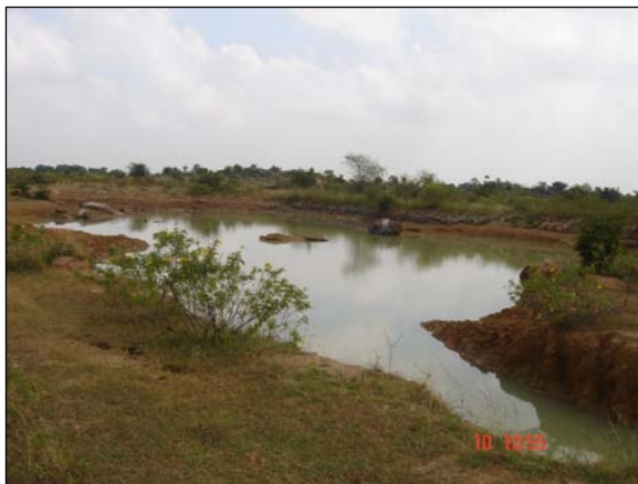
Picture 10. Percolation tanks constructed in the fallow land (left) and in the cultivated land (right) in the Irukodu watershed, Medak district.
