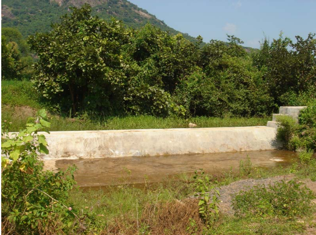
Picture 4. A surplus weir of a tank with quality construction in Chinnamallipuram
