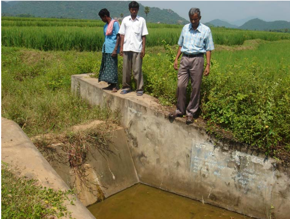
Picture 19. Check dam fully silted, however used as irrigation controlling drop structure for irrigating paddy crop.
