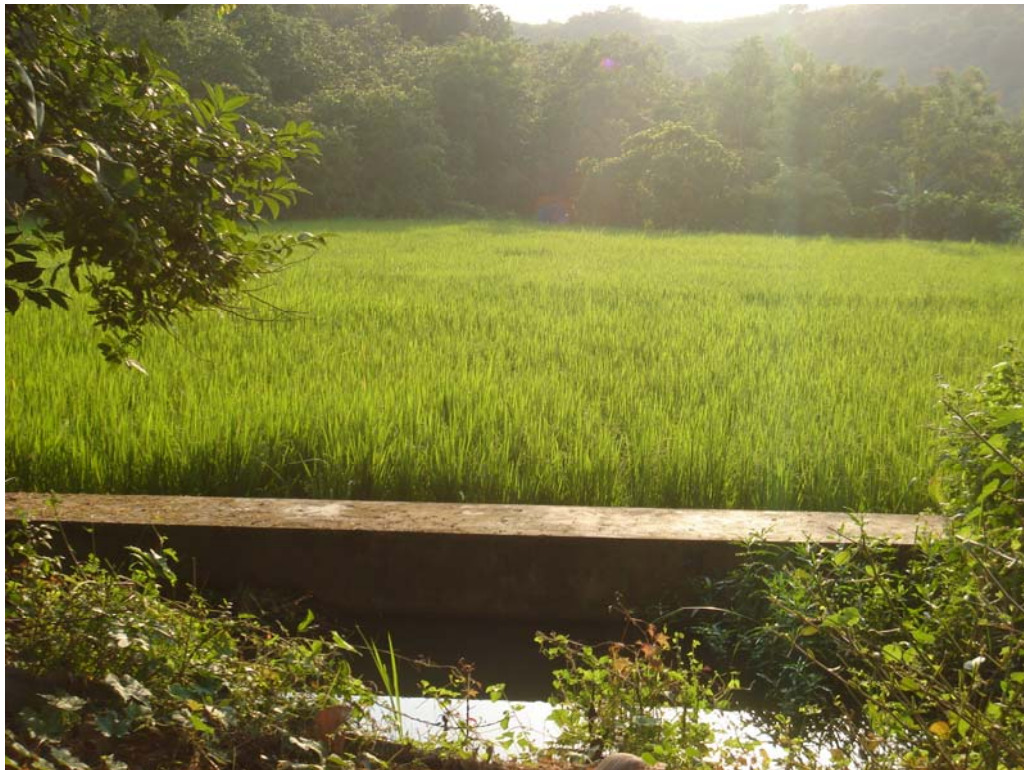
Picture 11. Silt protection/retention wall to protected bunds from erosion.
