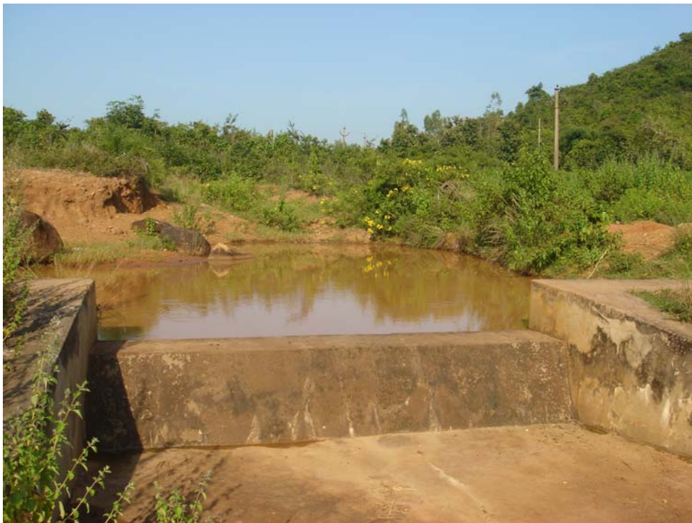
Picture 15. A masonry check dam with good storage of water, but no beneficiaries' fields around it.
