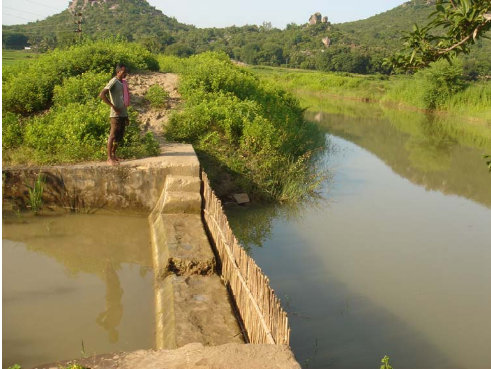
Picture 14. Renovated percolation tank with surplus weir in K. Mukundapuram used for fish culture and drinking water for cattle.
