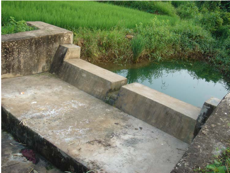
Picture 7. Good quality construction of a check dam in Degalapoluru WS, stored water used for irrigating paddy fields.
