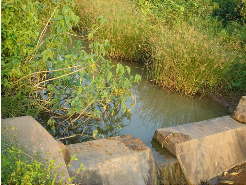
Picture 10. Masonry check dam with a notch to the body wall for dual purpose of control water flow for irrigation and storage in Ganguvada watershed.
