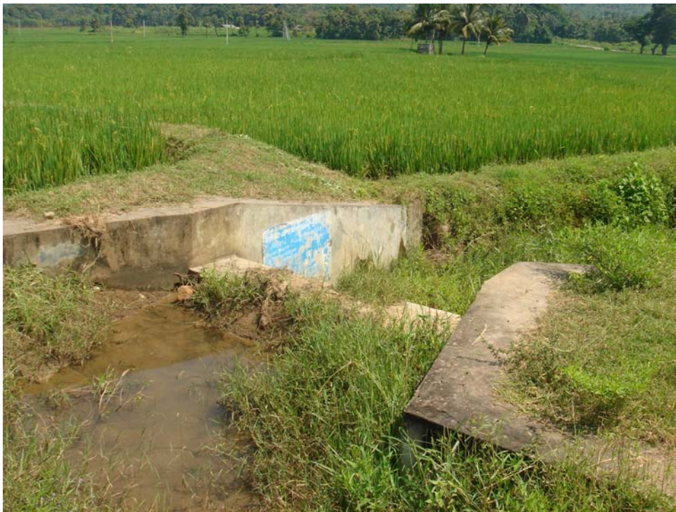
Picture 20. Check dams fully silted but used for controlling irrigation water to paddy fields in Sarvabonthu watershed.
