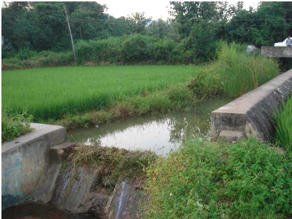
Picture 13. Silt protection wall of about 50 m length to protect breaching of field bunds in the nearby fields.
