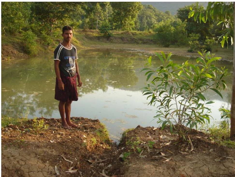
Picture 6. Renovated percolation tank with 0.5m height earthen bund in Degalapoluru ◆ The Check dam was in good condition and water is 1 ft below surplus weir. Water is used for irrigating paddy if necessary.
