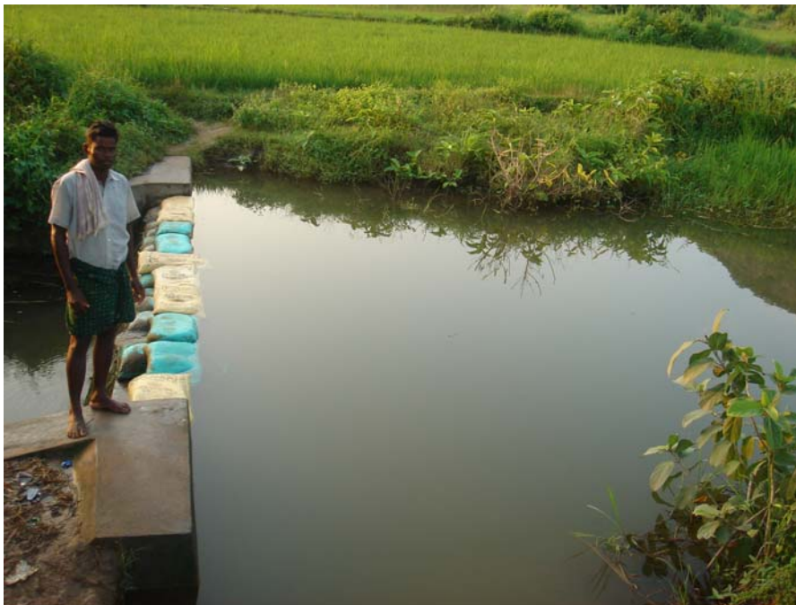
Picture 17. Lakshmi narayana check dam with 150 m 3 water storage capacity, enhanced storage by putting sand bags over it. 20 farmers benefitted on 100 acres paddy area.
