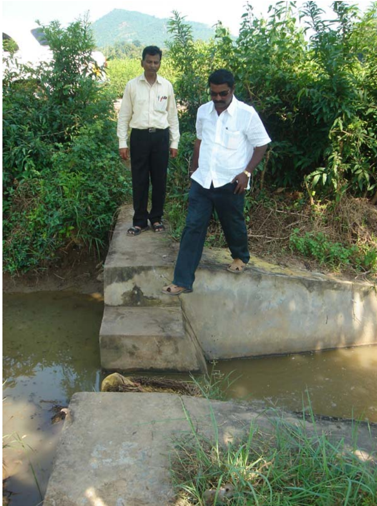
Picture 2. A drop structure in Burjawada used to irrigate fields around the drop by rising water level at the drop with an obstruction to notch.
