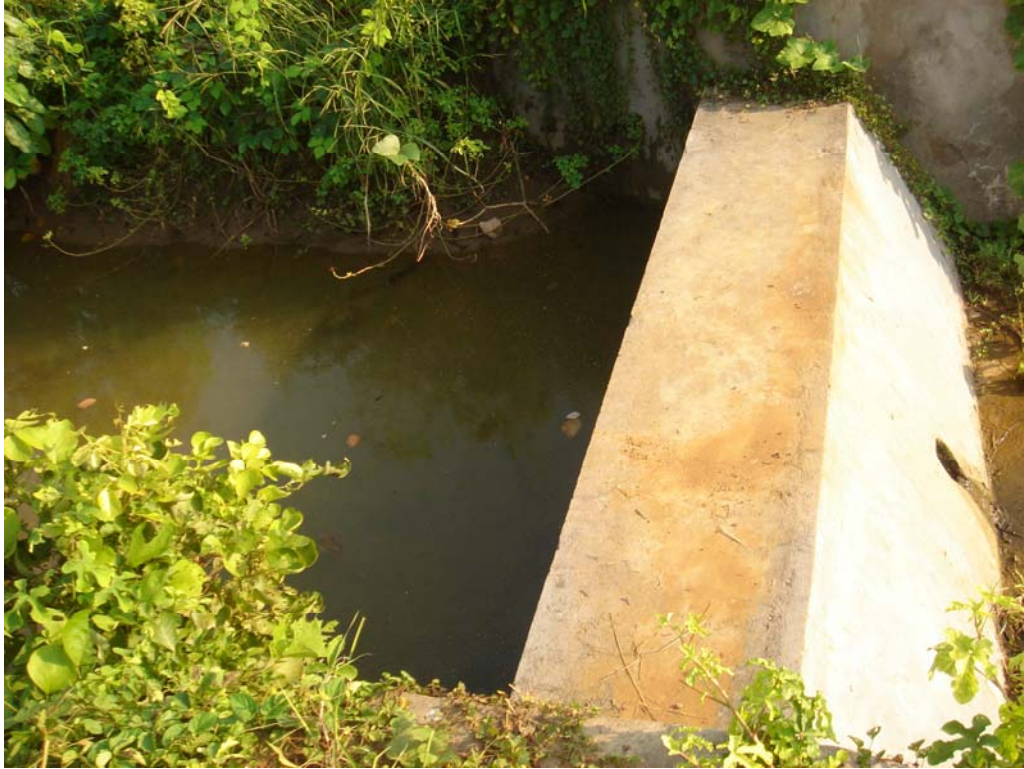
Picture 9. A check dam to store water for irrigation to paddy fields around and allow water down stream through a hole to check dam in Ganguvada watershed.
