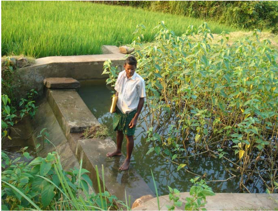
Picture 16. Appalam masonry check dam of 100m 3 storage capacity benefiting 6 farmers in 10 acres paddy fields.
