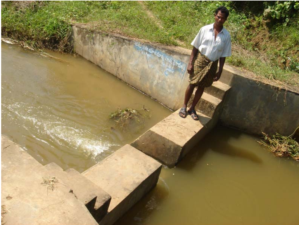
Picture 1. A drop structure on a deepened canal in Burjavadea used as irrigation canal rather than groundwater recharging check dam.
