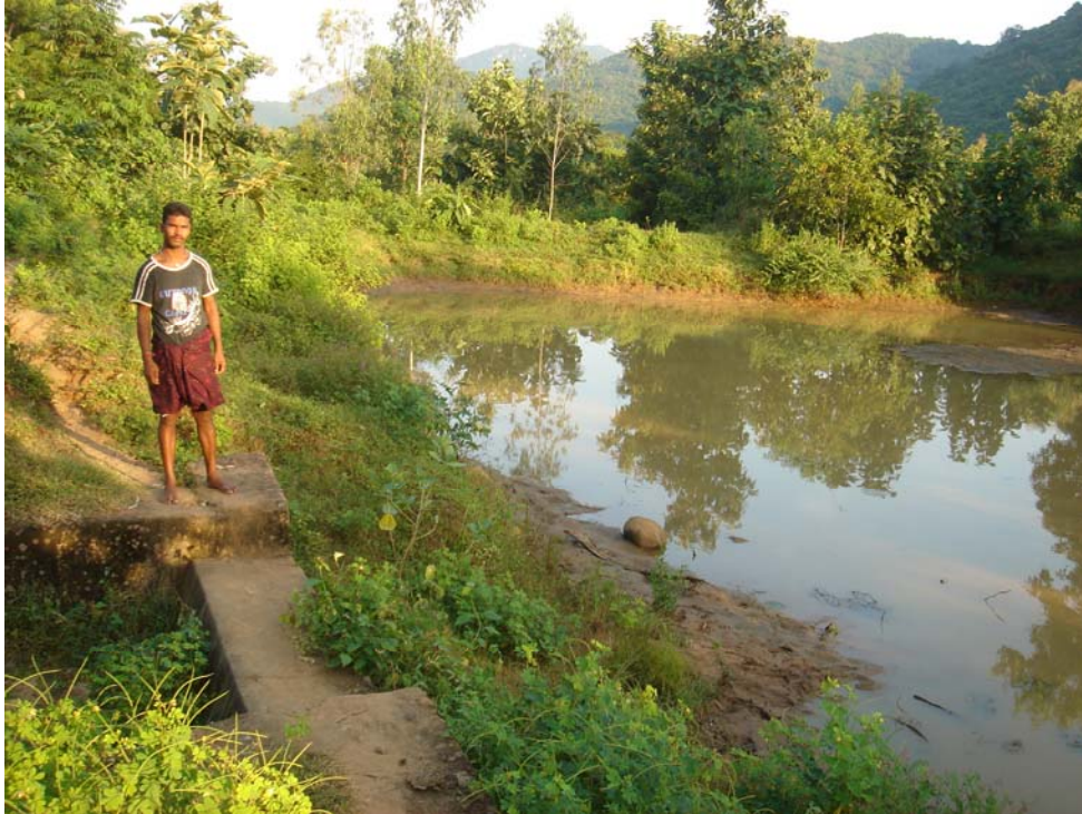
Picture 5. A renovated percolation tank with surplus weir in Degalapoluru ◆ Masonry check dam= 4 m width, 5Mt height, 10 m bunding (picture 7) having 1 feet storage at that point of time.
