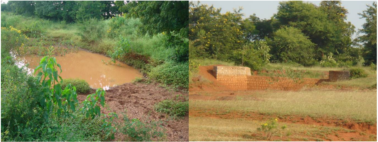
Fig: Sunken pit and check dam is supporting improvement in availability of water in wells and bore wells
