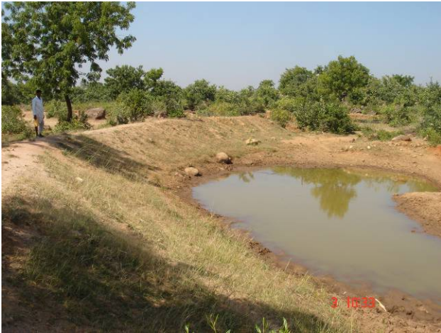
Fig: Percolation tanks with good water availability for ground water recharge
