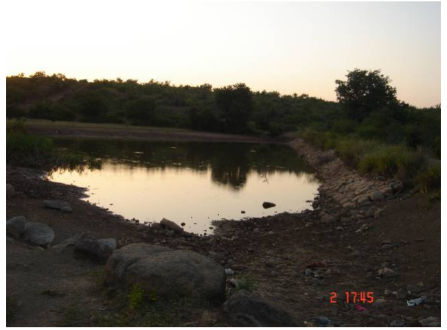
Fig: Check dam with full water stored and percolation tank with good water storage helped to recharge the ground water availability in wells and bore wells around the structure.
