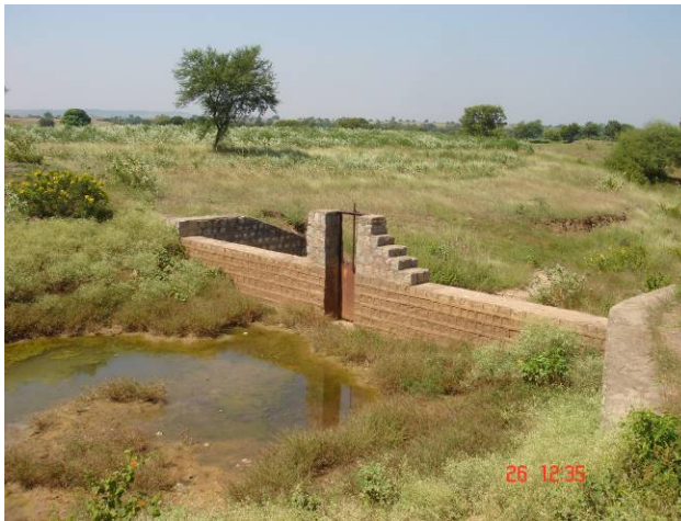
Fig: Focus group meeting with farmers and watershed committee members and a check dam with sluice gate which needs repair as leakage is there from bottom of the gate.
