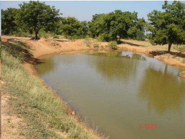
Fig: Percolation tanks with good water availability for ground water recharge
