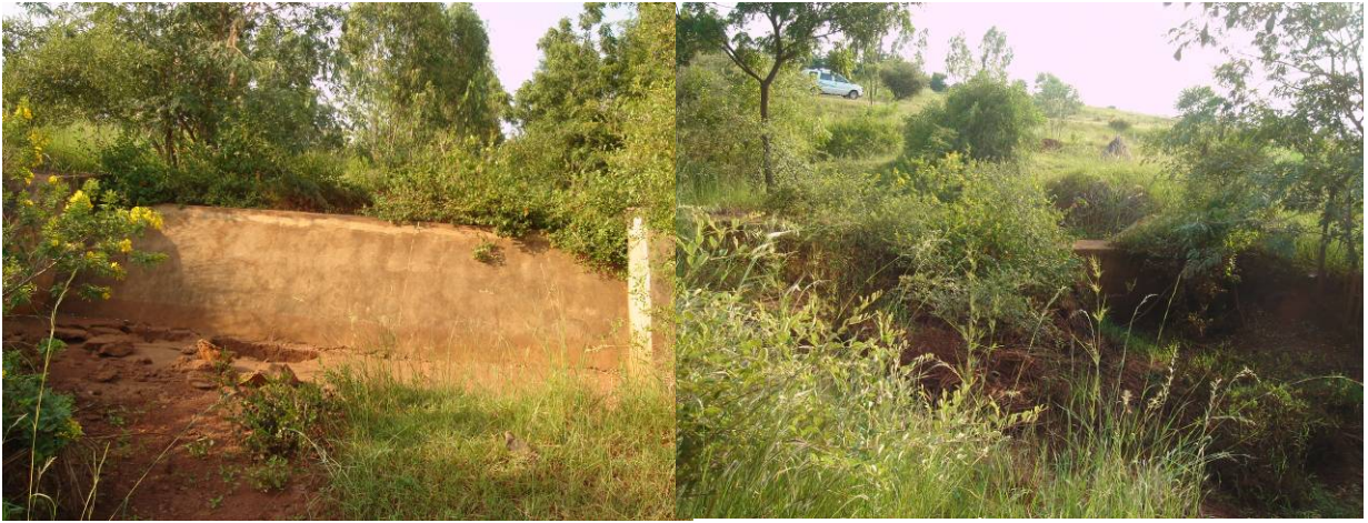
Fig: Masonry check dam apron damaged and full of silt plants and shrubs needs attention for better performance.
