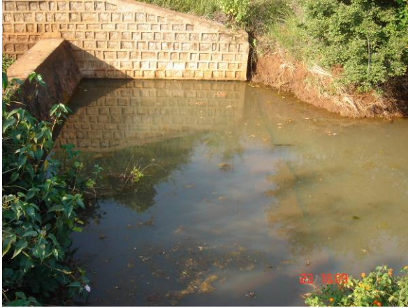
Fig: Check dam and percolation tank with good water stored for improved GWL in farmers wells and bore wells
