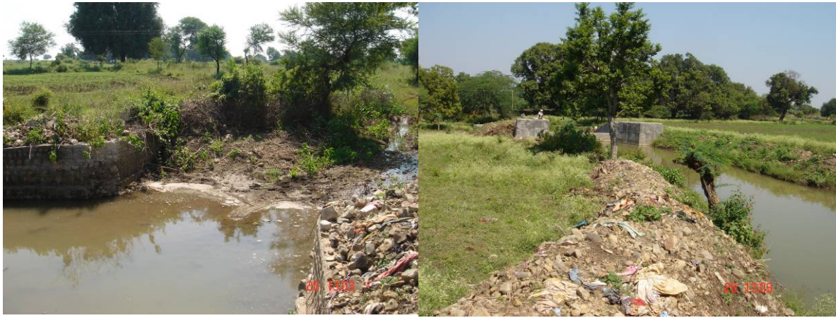
Fig: Check dam with full of water for ground water recharge and cattle drinking use
