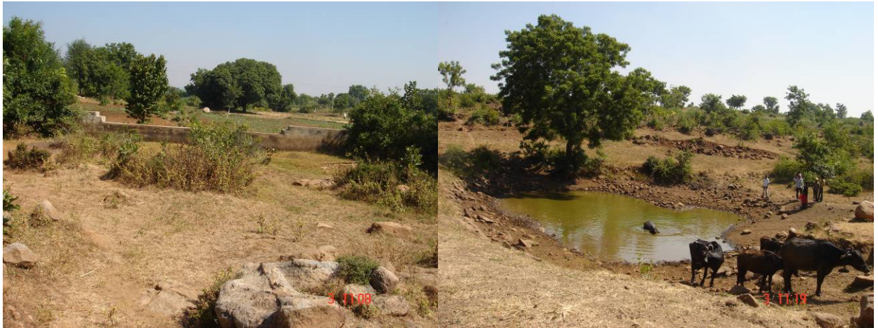
Fig: Percolation tank and check dam with good water availability for ground water recharge.
