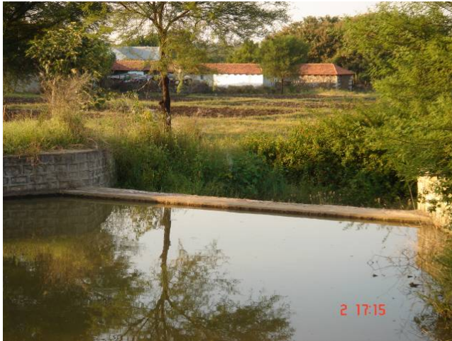
Fig: Check dam with full water stored and percolation tank with good water storage helped to recharge the ground water availability in wells and bore wells around the structure.
