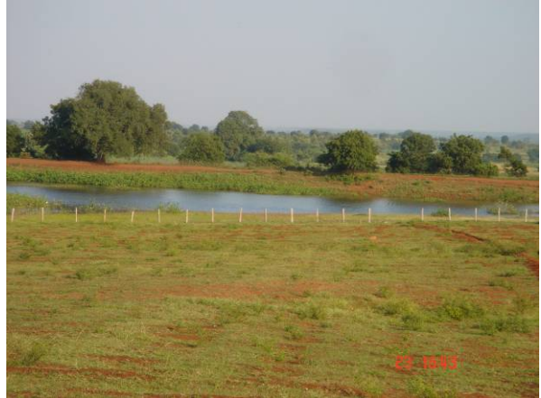
Fig: Check dam and percolation tank with good water stored for improved GWL in farmers wells and bore wells
