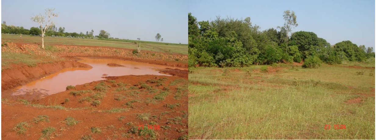
Fig: Percolation tank with siltation and plantation of teak and forest species in common land
