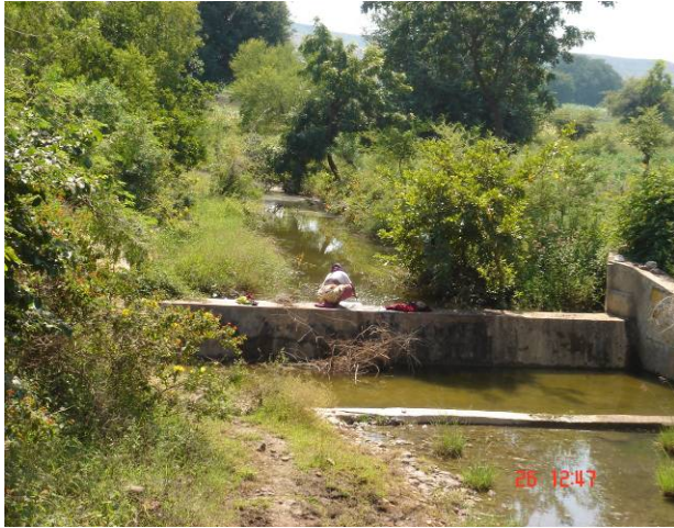
Fig: Check dam with full of water and percolation tank with deposition of silt and very little water.
