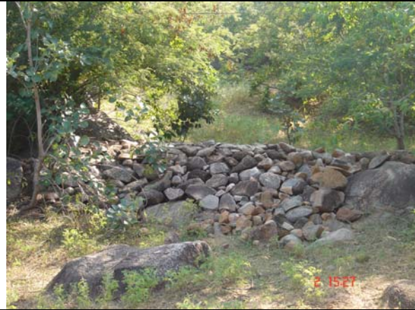
Picture 33. Damaged loose boulder structure in Sanjeevanraopet watershed.
