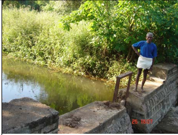
Picture 10. Masonry check dam with a gate to regulate the water release.
