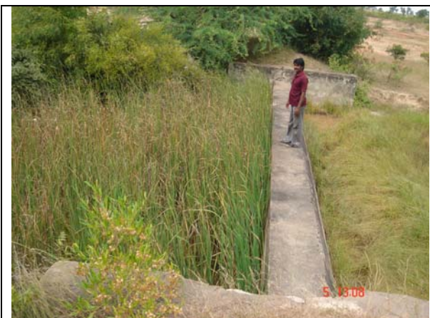
Picture 36. Masonry check dam in Regintala village, Medak district.
