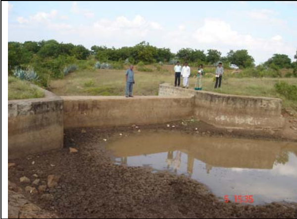
Picture 15. Masonry check dam with stored water and silt accumulation in Maddikunta watershed.
