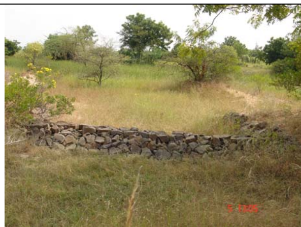
Picture 37. Loose boulder structure in Regintala village, Medak district.
