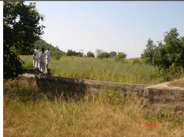
Picture 19. Masonry check dam in the Masanapally watershed.
