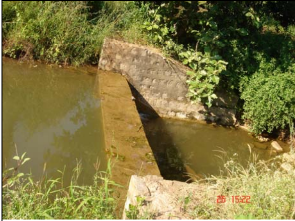
Picture 7. Check dam with full of water in Edulapally watershed.
