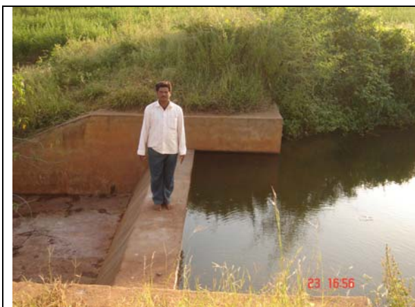
Picture 29. Masonry check dam in the Sajjaraopet watershed.
