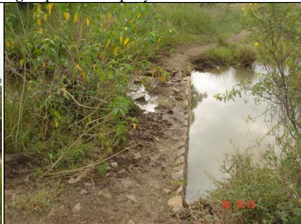
Picture 4. A check wall across a drain to store water and people to cross over it.
