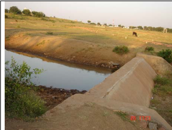
Picture 5. A masonry check dam in Budera watershed along with converted land in to residential plots.
