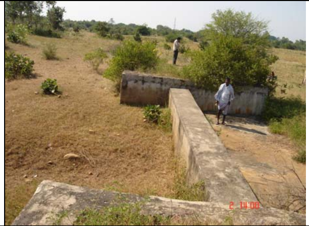
Picture 26. Masonry check dam in the Rayalamadugu watershed.
