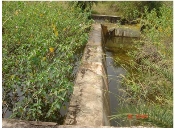
Picture 12. Masonry check dam with overflowing water and grown up bushes in Gadipeddapur watershed.
