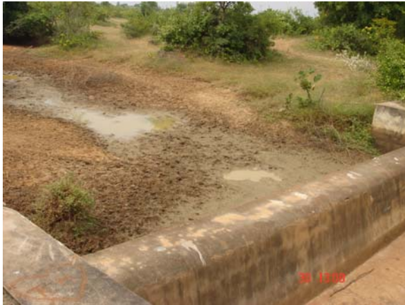
Picture 11. Masonry check dam with accumulated silt in Gadipeddapur watershed.
