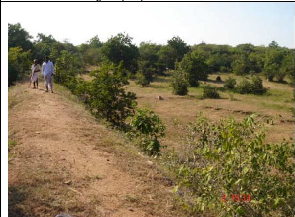
Picture 34. Percolation tank constructed in fallow land in Sanjeevanraopet watershed.
