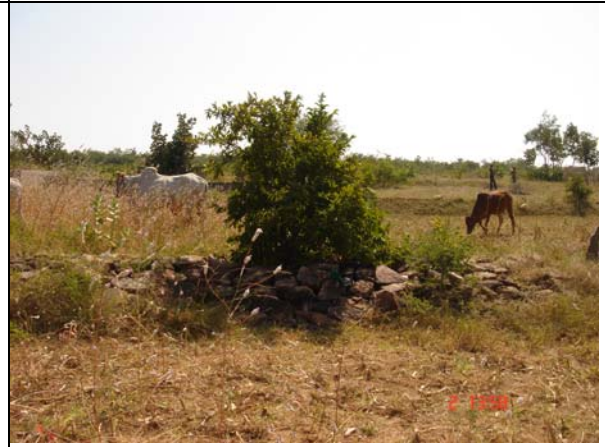
Picture 28. Condition of rock fill dam in the Rayalamadugu watershed.
