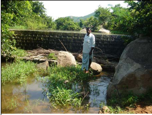
Picture 1. Good quality check dam in Abangapatnam needs apron repairs.
