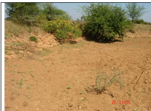
Picture 3. Big percolation tank in Allapur requires desilting for improved storage.
