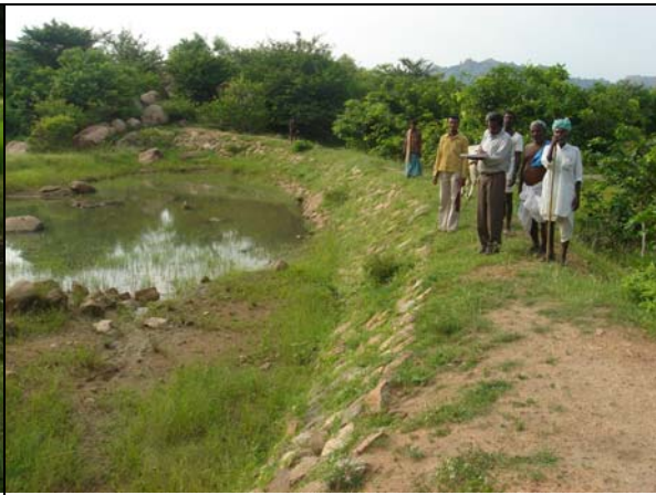
Picture 6. Big percolation tank in Azilapur requires desilting, strengthening of bund
