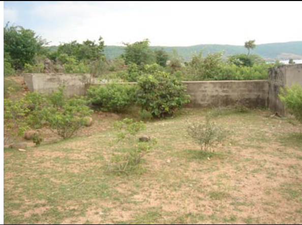
Picture 23. Check dam silted up and requires bush cleaning in Malleswaram
