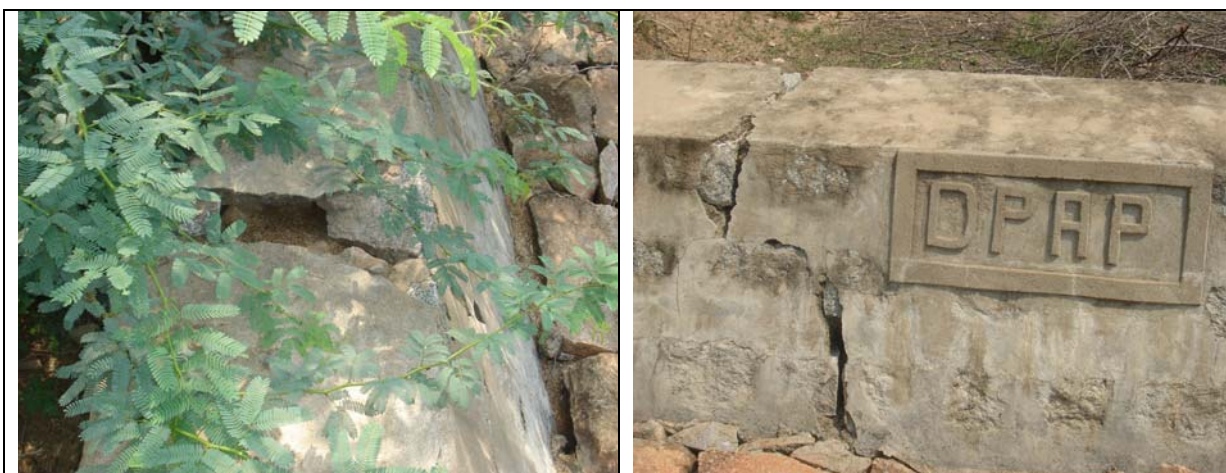
Picture 13. A check dam with cracks developed at Madigolla manyam in Janumpally.
