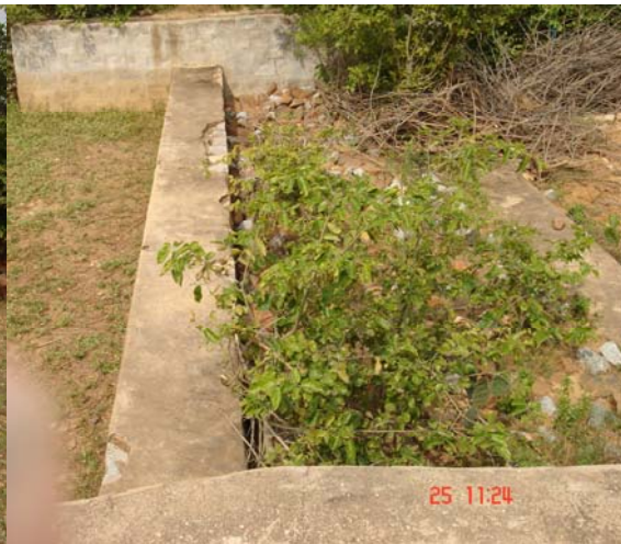
Picture 27. Check dam silted up and requires maintenance in Mannapur
