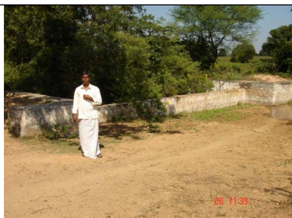
Picture 4. Check dam requires desilting, closer of breaches to side walls in Allapur.
