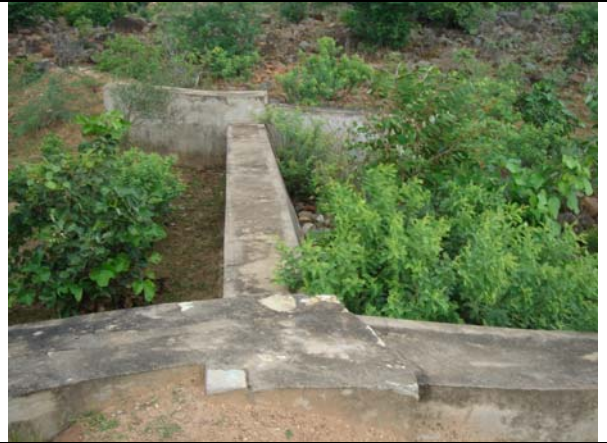
Picture 24. Check dam with bushes around it requires bush cleaning in Malleswaram.
