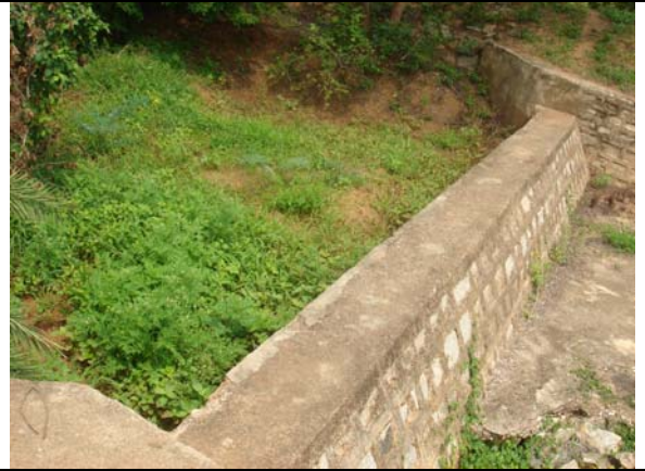
Picture 12. Leakages were found for a check dam but no repairs were undertaken in Jamisthapur.
