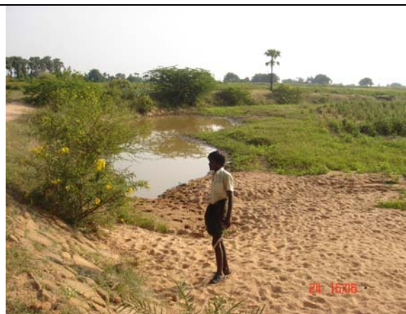
Picture 30. Percolation tank silted up after the floods in 2009
