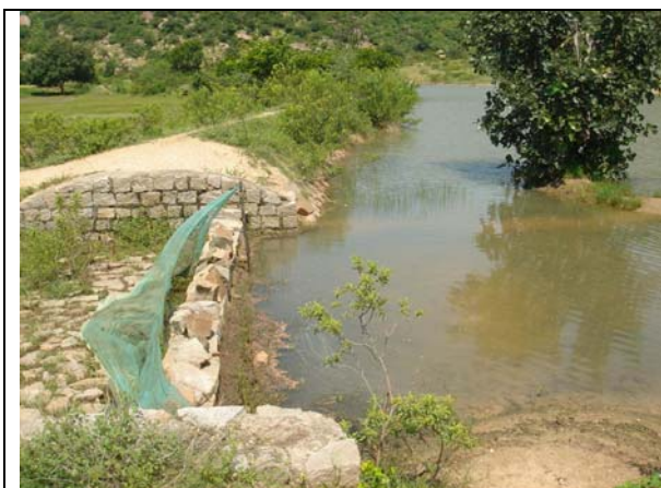
Picture 17. A percolation tank with good storage and a spillway, but silted up
