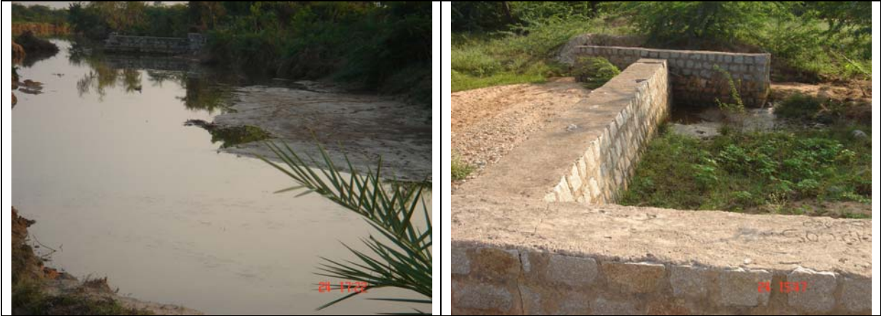
Picture 6. In Eklaspur all watershed structures were damaged after devastating floods during October 2009 in Mahabubnagar.
