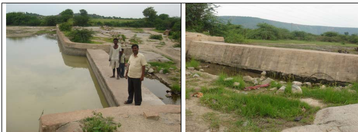
Picture 12ab. Check dams in Inole watershed in Achampeta mandal constructed under DPAP-1.
