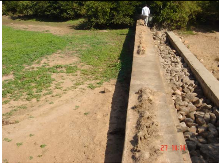
Picture 5b. Check dam across Kondareddy Palli cheruvu vagu Chinnarevally needs filling up of stone packing of apron.
