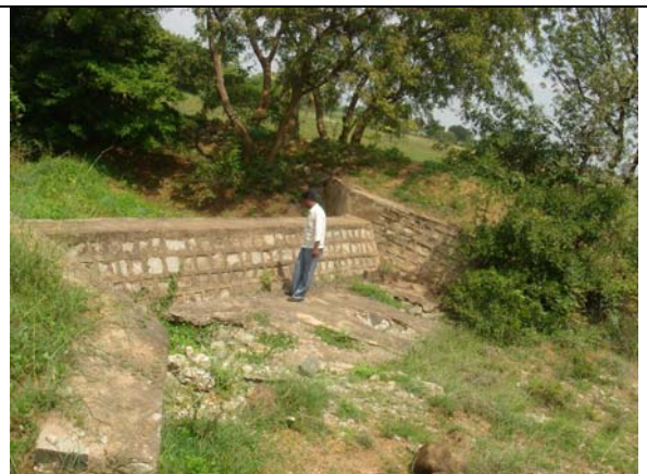
Picture 4b. A check dam in Boypally with breaches to the apron.
