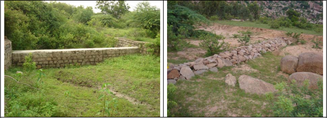
Picture 3. Check dam and Loose Boulder structures in Bollaram watershed under DPAP-1.
