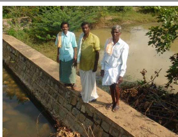
Picture 7b. A check dam with breaching near the side wall.
