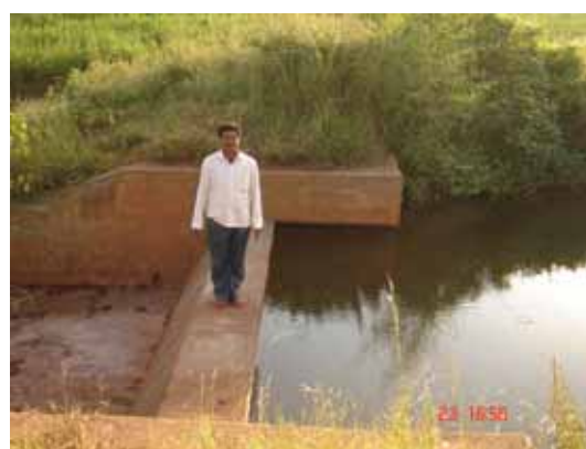
Figure 2. Check dam at Sri Sai watershed.
