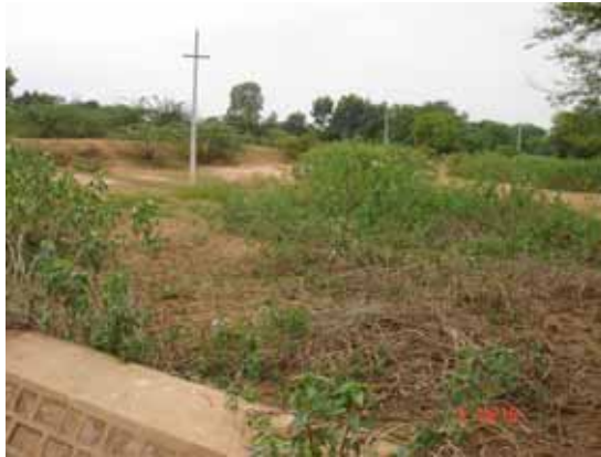
Figure 3. Check dam filled with sediment and bushes at Sri Sai watershed.
