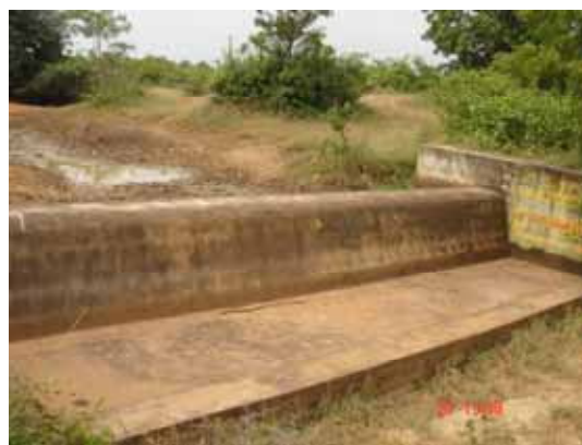
Figure 2. Check dam at Pragathi watershed.
