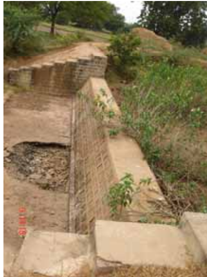
Figure 3. Check dam filled with sediment, bushes and damage on apron at Dandumaisamma watershed.
