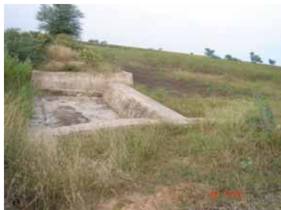
Figure 2. Check dam at Brahma watershed.
