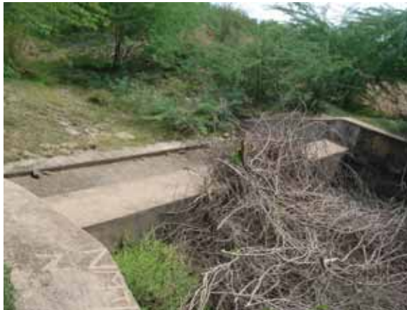
Figure 3. Check dam filled with sediment and bushes in Chennakeshava watershed.
