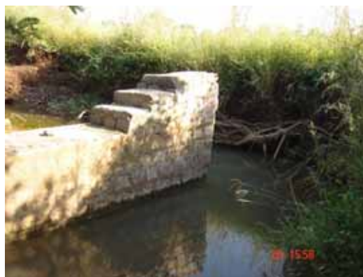
Figure 3. Incomplete check dam serving no purpose at Dirisanapally watershed.
