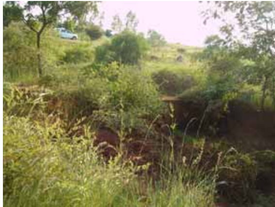
Figure 3. Check dam filled with sediment and bushes at Jillepally watershed.
