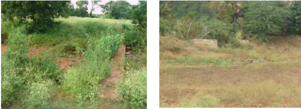
Figure 3. Check dam and percolation tank filled with sediment and bushes, Muthyalamma watershed
