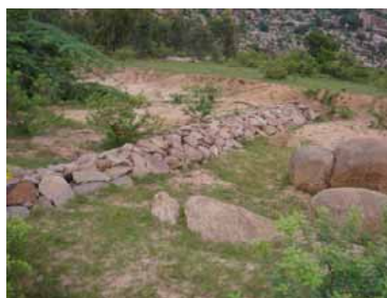
Figure 2. Rock fill dam at Pogilla watershed.
