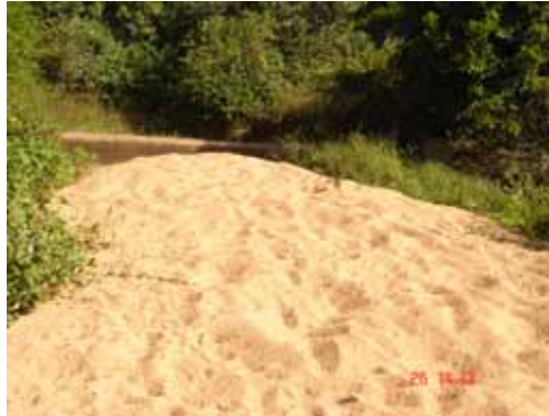
Figure 3. Check dam filled with sand and bushes at Brahma watershed.
