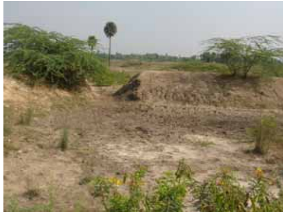
Figure 3. Damaged percolation tank at Pragathi watershed.
