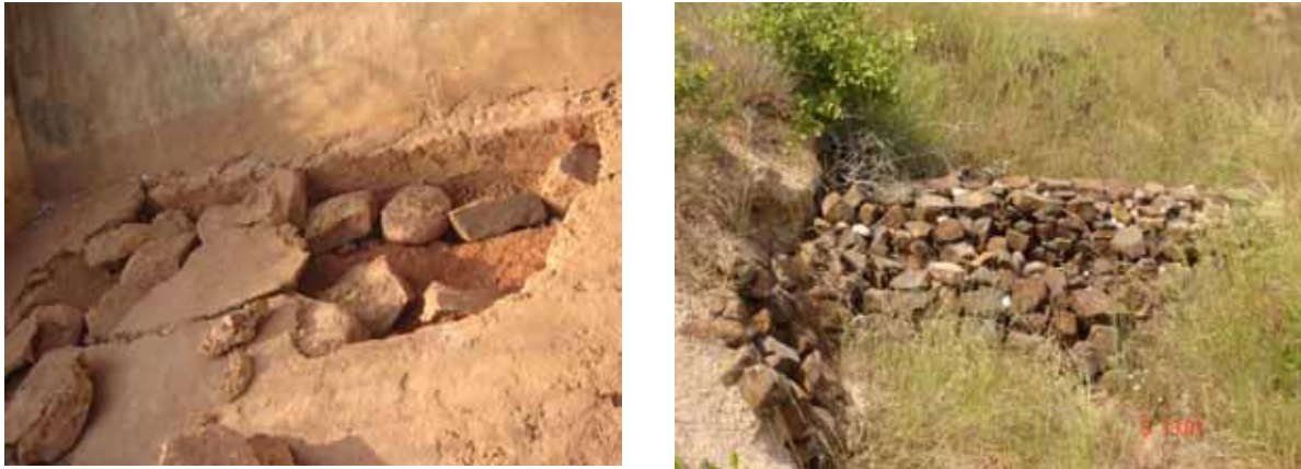
Figure 3. Damaged apron wall of check dam (left) and rock fill dam (right) in Chamuledu watershed.
