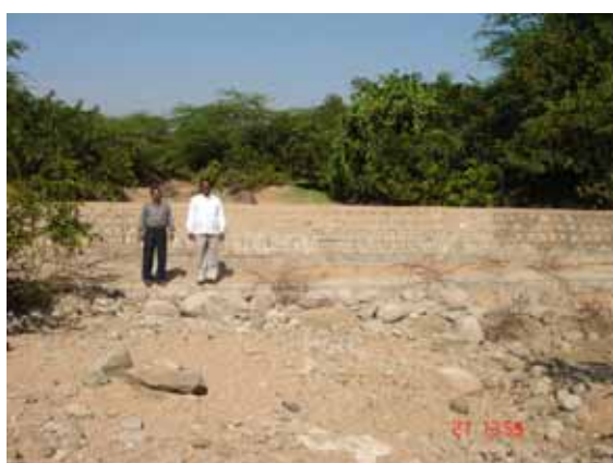
Figure 1. Check dam at Pogilla watershed.
