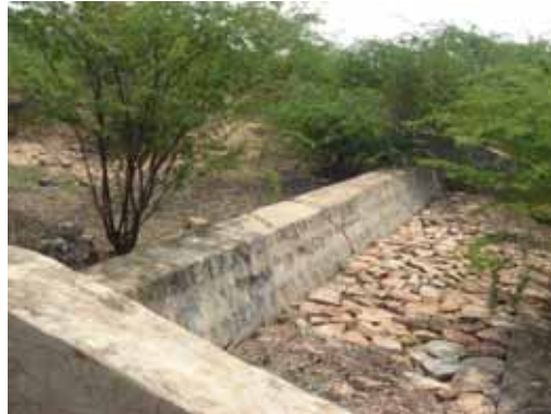
Figure 3. Check dam filled with sediment and bushes at Kranthi watershed.
