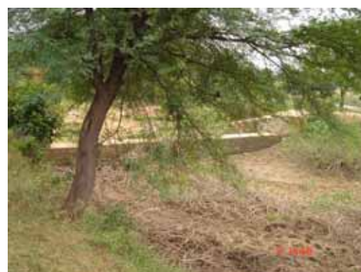
Figure 2. Check dam at Jillepally watershed.
