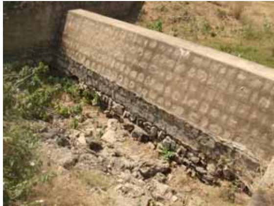
Figure 3. Damaged apron wall of check dam in Annadata watershed.
