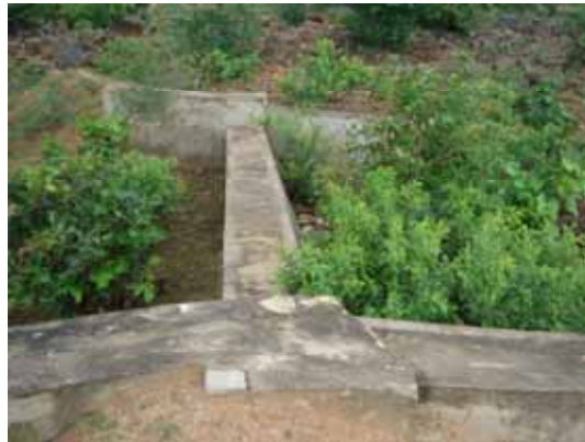
Figure 3. Check dam filled with bushes at Tallasingaram watershed.
