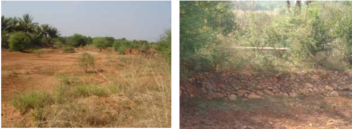
Figure 3. Percolation tank and spillway filled with sediment and bushes, Krishna watershed
