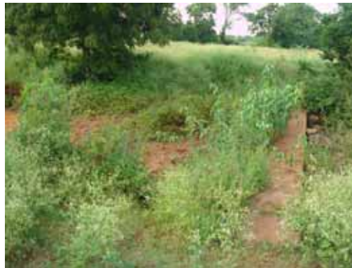
Figure 3. Check dam filled with sediment in Anjaneya Swamy watershed.
