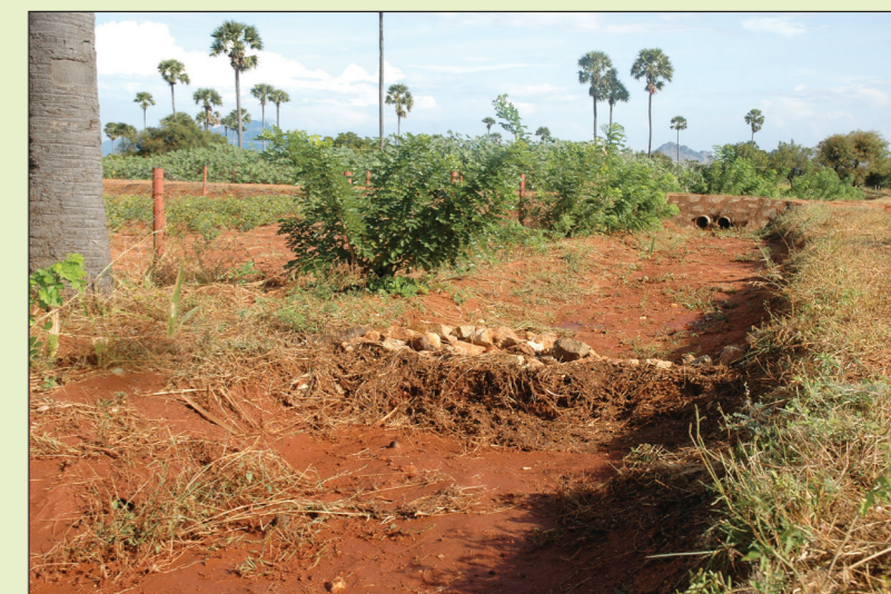
Rock earth dams convert gullies into reservoirs.
