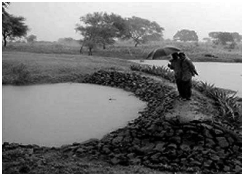
FIGURE 5 Water-harvesting structure in Adarsha watershed Kothapally, Andhra Pradesh.
