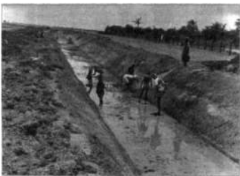
Construction of main drain.
