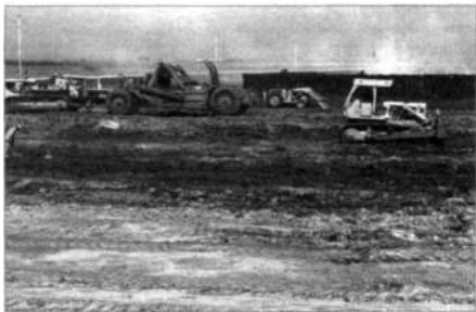
Field under development.
