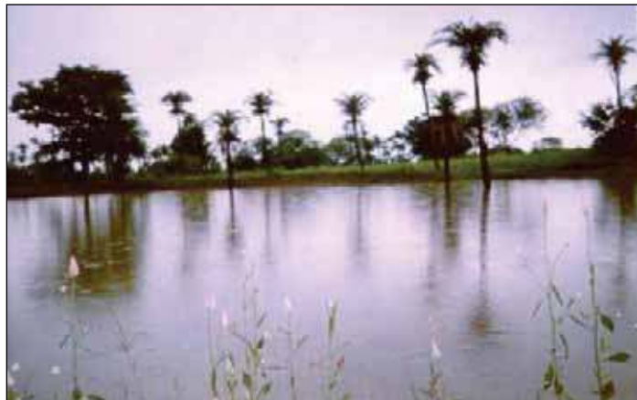
Fig. 11. Earthen check dam at Lalatora watershed, Vidisha, Madhya Pradesh.
