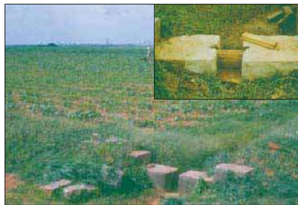
Figure 5. Gated-outlet contour bund with water stagnation (gated-outlets are shown in inset).
