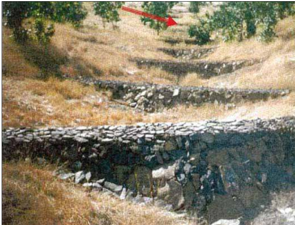
Figure 14. Series of loose boulder wall gully checks at Bundi watershed, Rajasthan.
