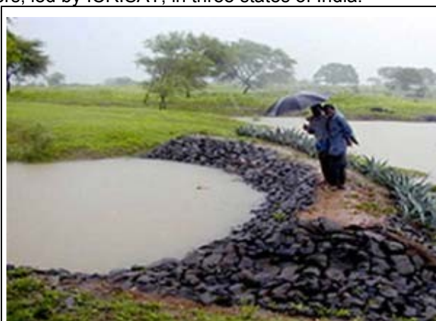
Low-cost mini-percolation tank (earthen structure) at Kothapally watershed, Andhra Pradesh.
