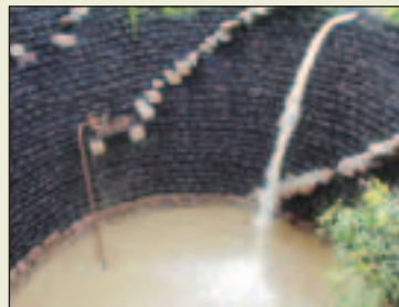
Well recharging with runoff water.
