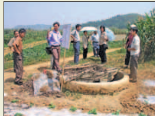
Underground tanks/cisterns for harvesting run-off in Xiaoxingcun watershed, China.
