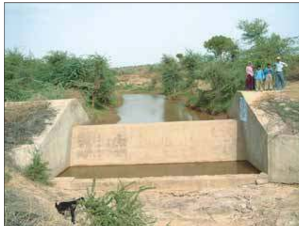
Figure 19. Masonry check-dam for controlling gully and recharging groundwater in Bundi, Rajasthan, India.
