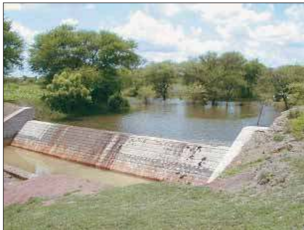
Figure 18. Masonry check-dam for controlling gully and water harvesting in Adarsha watershed, Kothapally, Andhra Pradesh, India.
