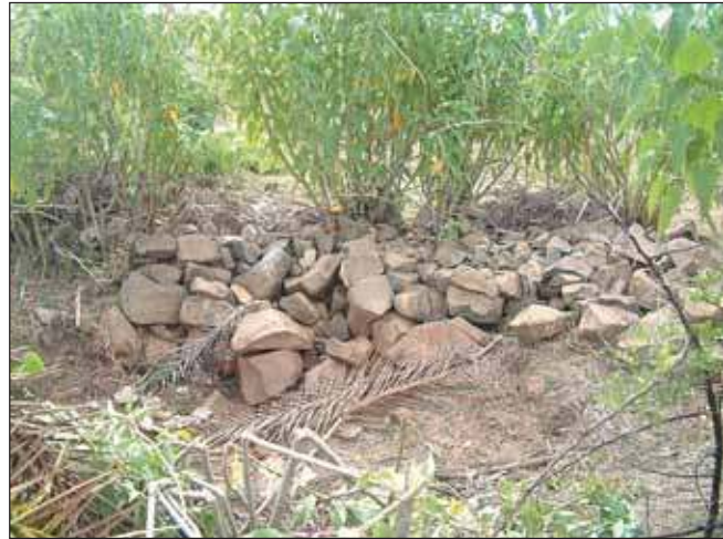
Figure 7. Loose boulder check with shrubs for controlling small gully.
