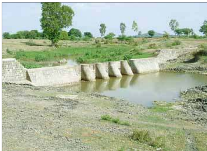
Figure 20. Masonry check-dam with additional support for stability in Madhusudhangadh watershed, Madhya Pradesh, India.
