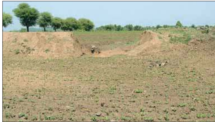
Figure 2. Improper land development leads to damage of structure and gully formation as in Madhusudhangadh, Madhya Pradesh, India.
