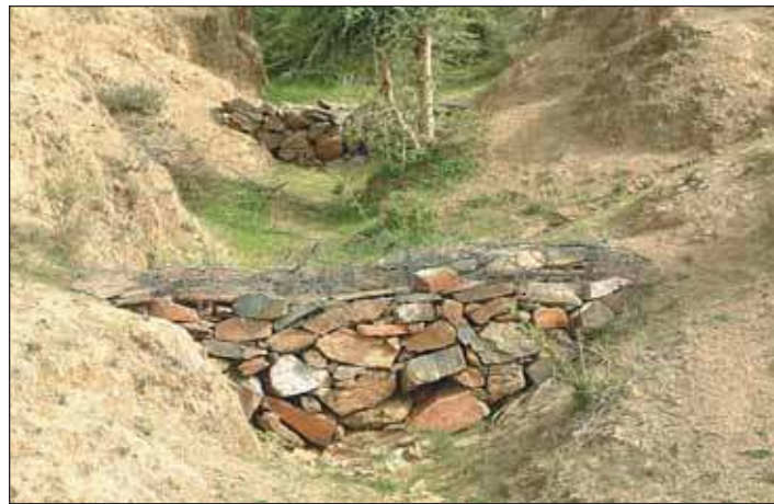
Figure 17. Series of stone wall dams for controlling gully in Bundi, Rajasthan, India.
