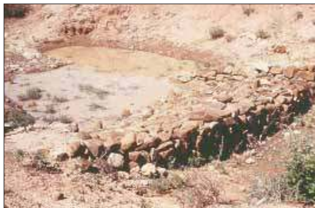
Figure 10. Loose rock drop structure for controlling gully erosion in Mittimari watershed, Karnataka, India.
