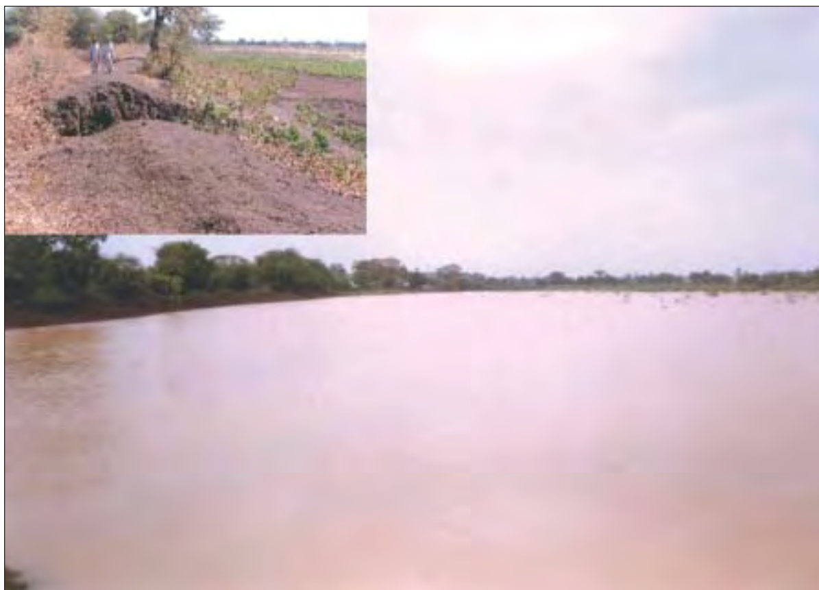
Figure 5. Water storage in the renovated big pond in Ringnodia micro-watershed after the first major runoff event in June 2001.
