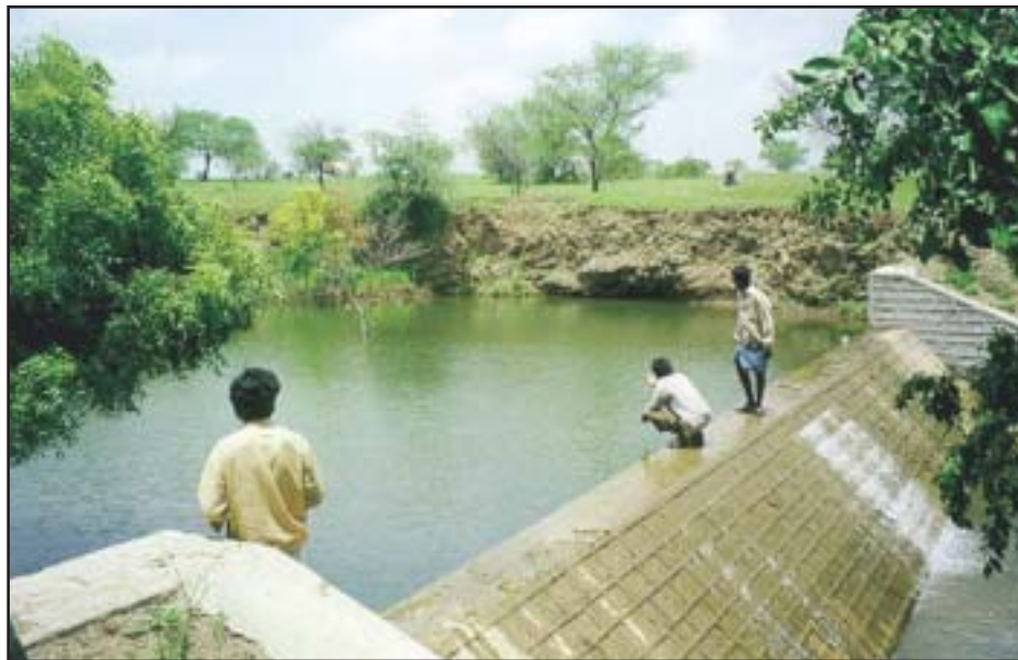
Figure 2. Community-based masonry check-dam.
