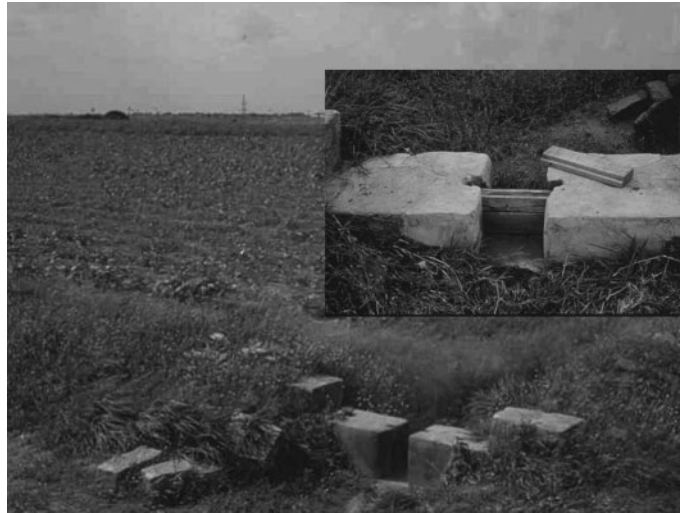
Figure 7.10 Gated-outlet contour bund system at ICRISAT, Patancheru, India; (inset) gated-outlet
