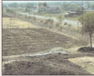
Boundary fence installed by the project at Jalgaon Oilseeds Research Station, Maharashtra, India.
