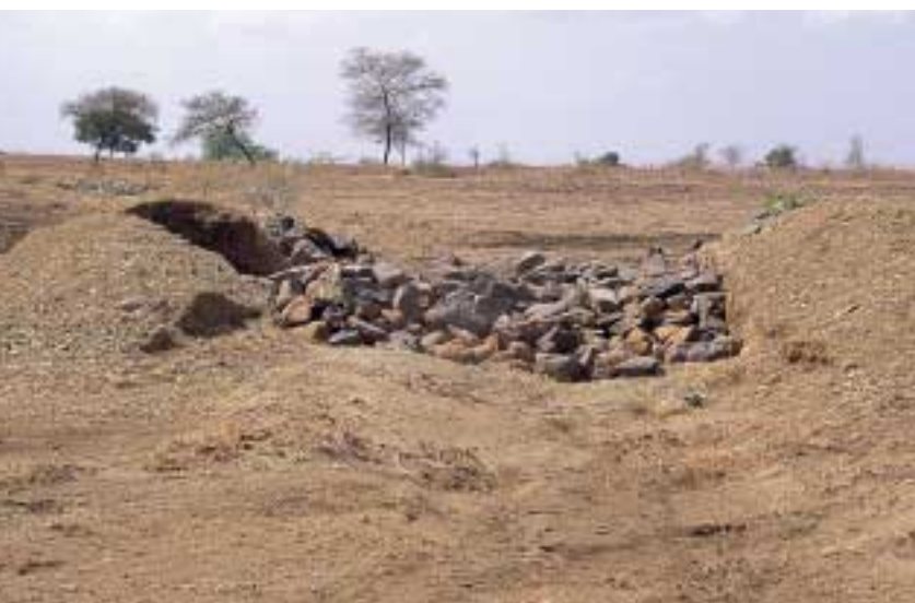
Rock / earth dams convert gullies into reservoirs
