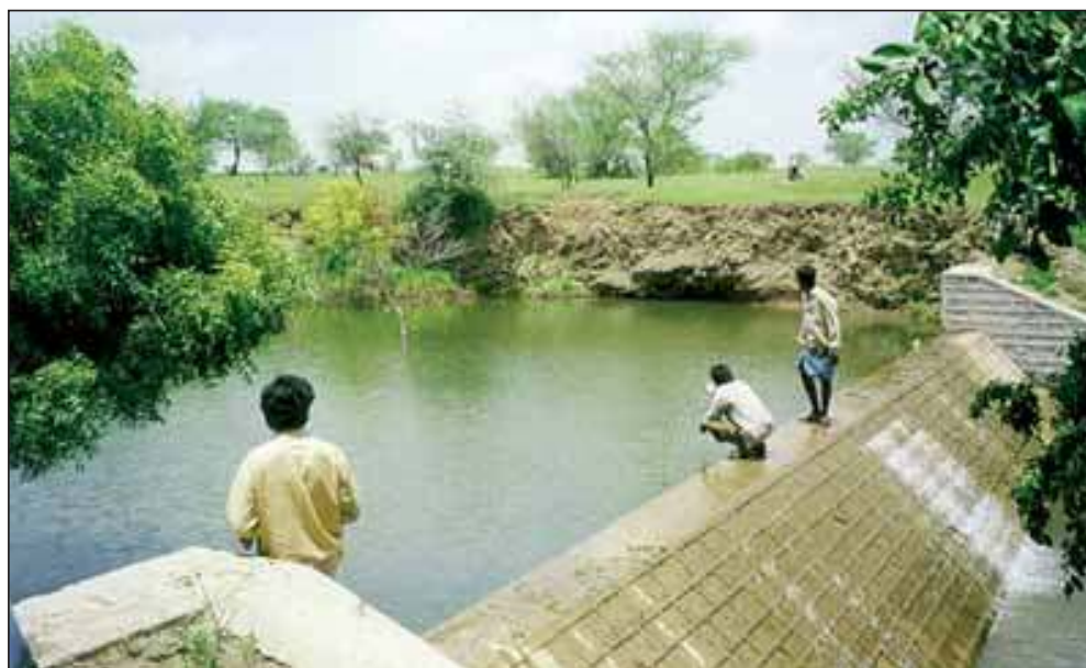
Figure 5. Community-based masonry check dam.
