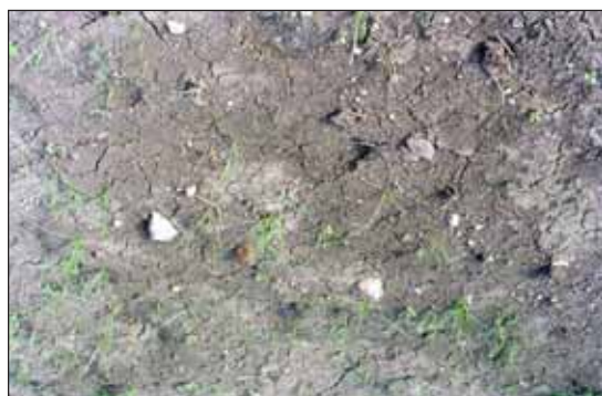
(b) More than 0.5 cm polygonal cracks on the surface of Nipani soil.
