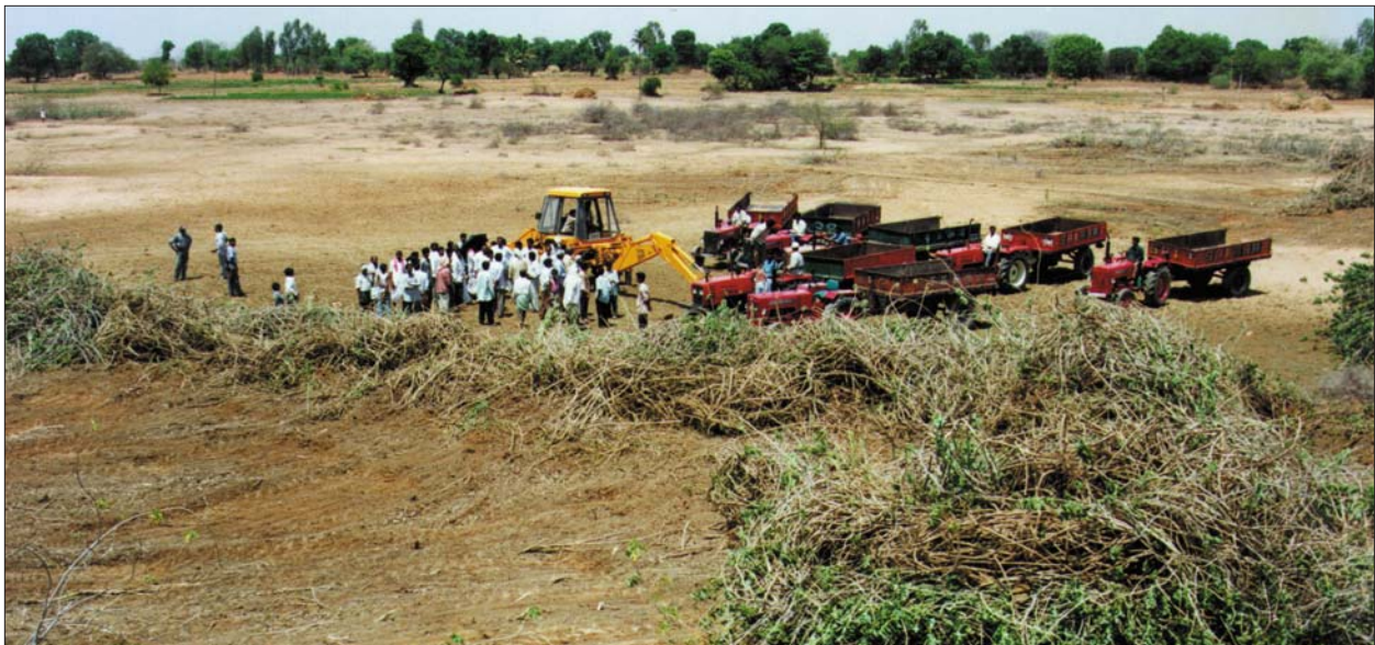
Fig 1. Desilting work at Reddykunta tank, Wargal mandal, Medak district.
