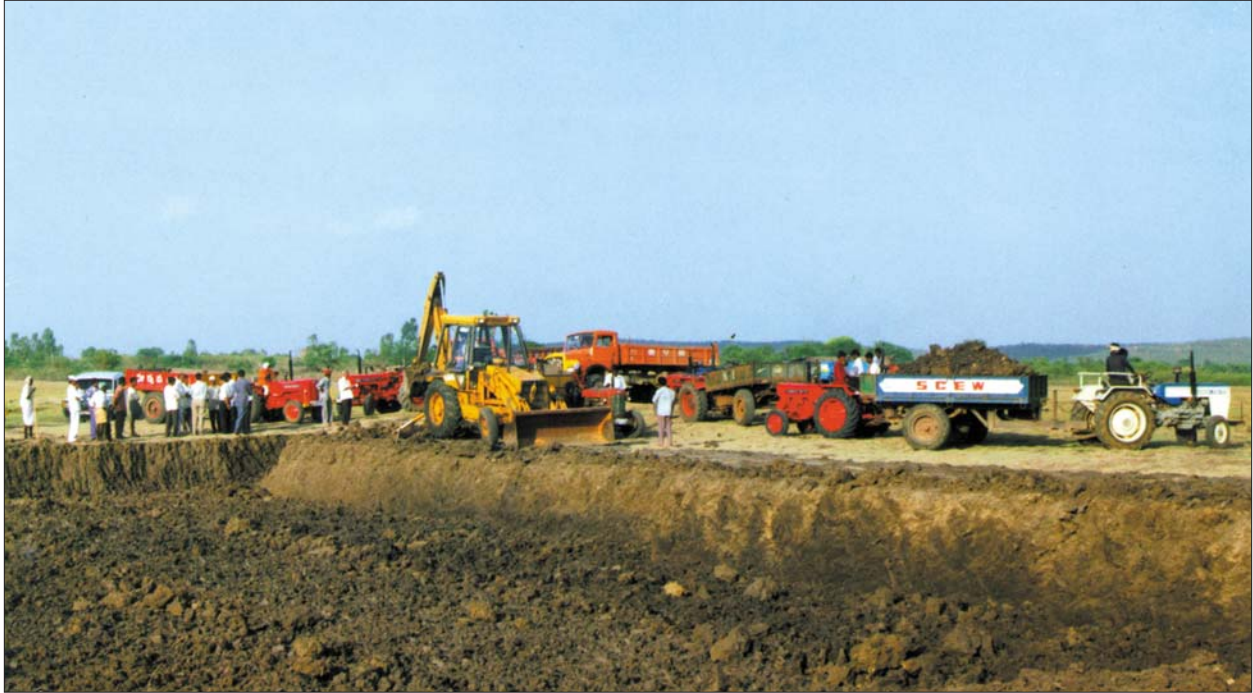
Fig 4. Desilting work by digger at Peddacheruvu tank, Narsapur mandal, Medak district.
