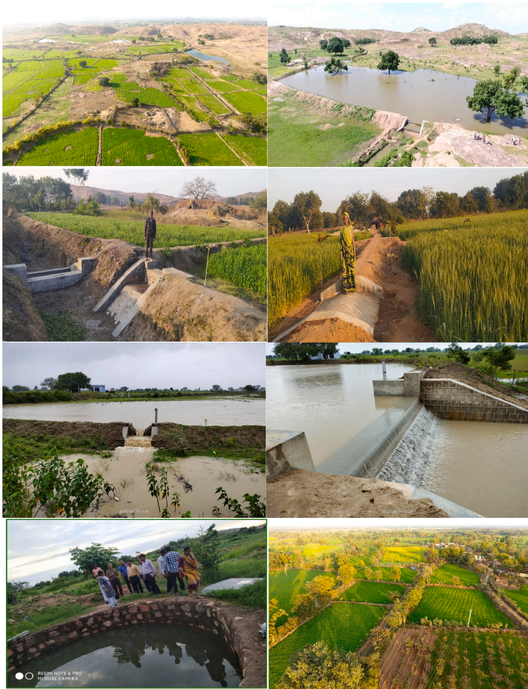
Fig. 2. Selected images of landscape resource conservation interventions, runoff monitoring stations, groundwater well, and cultivated crops in the study area; Panel 1 (left): Drone view of the study area showing constructed water bodies at the foothills, diversion drains, and field bunding; Panel 1 (right): Zoomed-in view of the first rainwater-harvesting structure constructed at the foothill; Panel 2 (left and right): Zoomed-in views of field bunds with masonry surplus structures; Panel 3 (left and right): Hydrologic monitoring systems at field (S3) and reservoir outlet (S1); Panel 4 (left): Dug well with elevated water table in October 2022; Panel 4 (right): Aerial view of the study area with crops during the rabi season in 2022.
