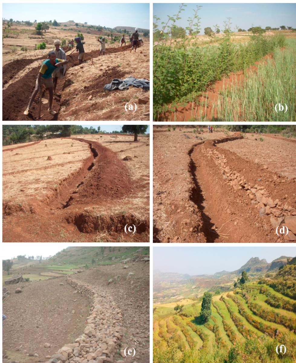
Fig. 6. Pictures of commonly applied land management practices: a) graded soil bund (ditches on upper side to discharge runoff), b) graded soil bund with vegetative hedgerows, c) graded fanya juu (ditches on lower side), d) stone faced soil bund, e) stone terrace, and f) bench terrace.
