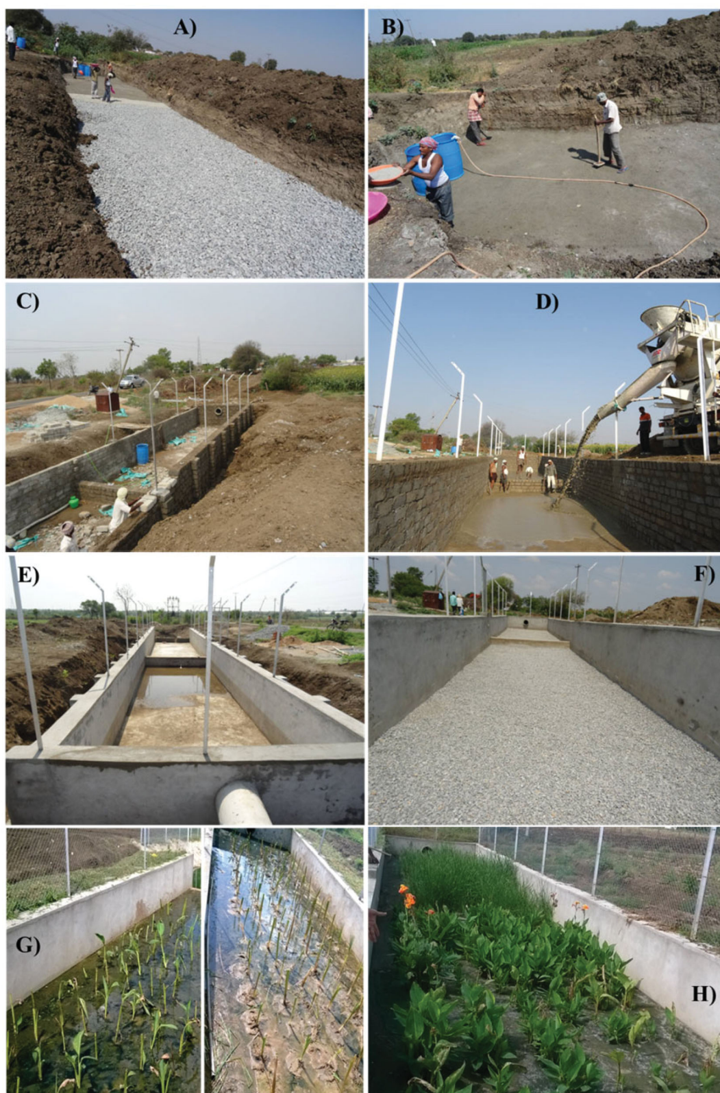
Figure 2. Different phases of construction of the constructed wetland; bed preparation (A), compaction (B), masonry work (C), introduction of concrete liner (D), completion of plastering and curing (E), filling-up of the filter media constituents (F), plantation (G), stabilization (H).
