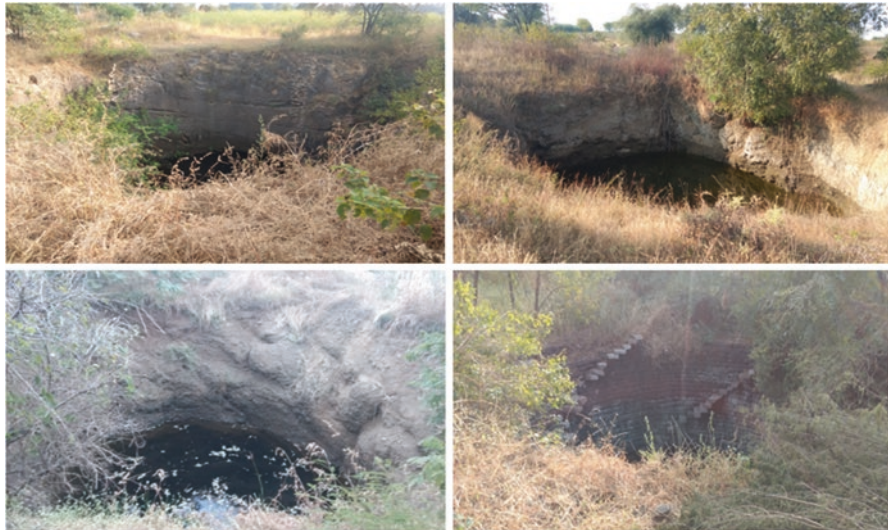
Fig. 8.26 Unused open wells in Kothapally
