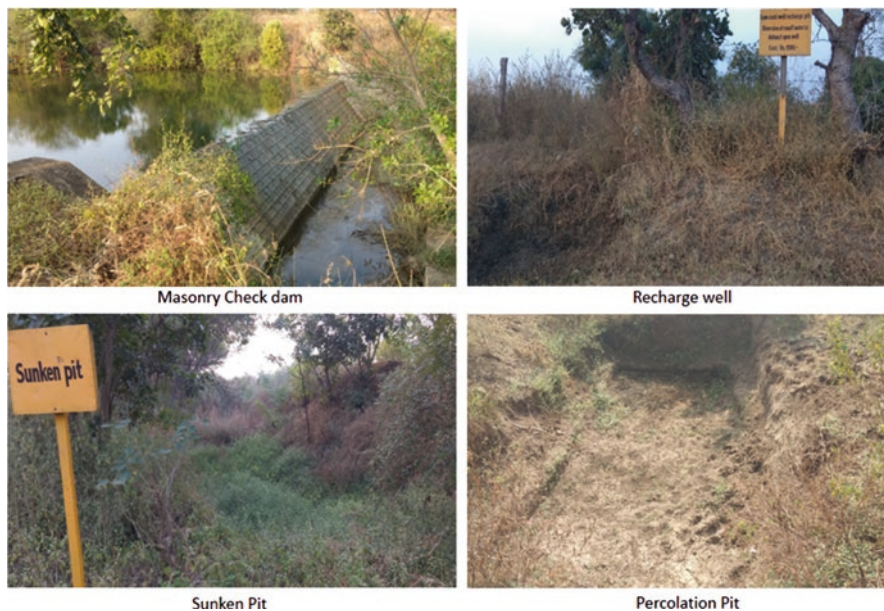
Fig. 8.28 Rainwater harnessing structures in Kothapally
