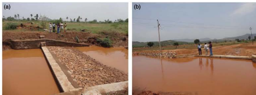
Fig. 4.20. Check-dam full with rainwater in (a) Kodalu and (b) Chikanthapur villages.
