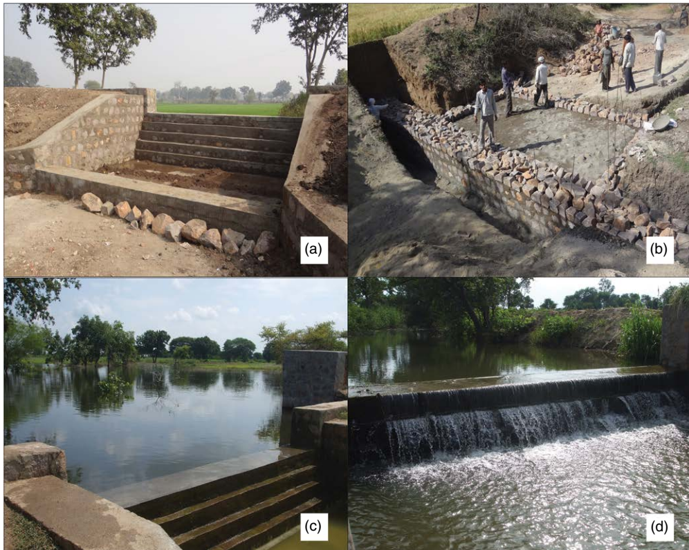
Fig. 7.5. Rainwater harvesting in watershed: (a, b) check-dams constructed at different locations; and (c, d) water harvested in check-dams during the rainy season 2013–14.
