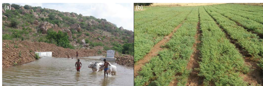
Fig. 10.2. In-situ and ex-situ soil and water management interventions implemented at POWERGRID–ICRISAT watersheds: (a) check-dam at Bugganipalli, Bethamcherla, Kurnool; (b) broad-bed and furrow system at Ukkali, Vijayapura.
