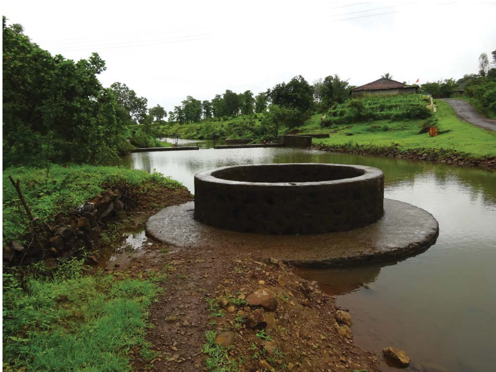
Fig. 4.8. Desilted check-dam in Kogda village.
