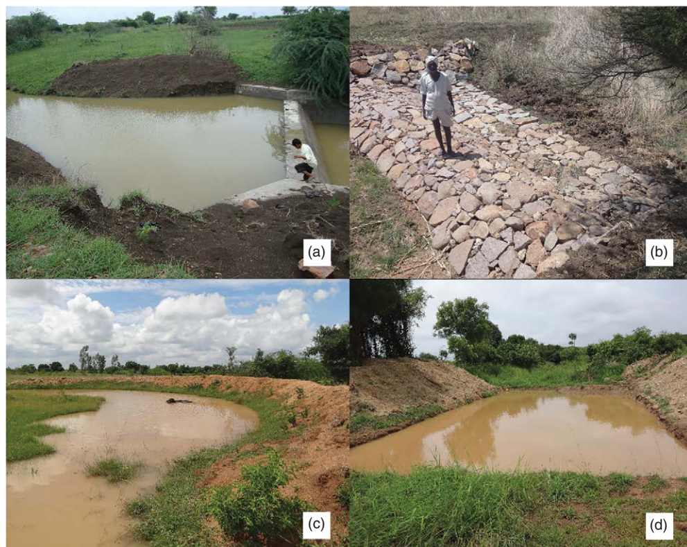
Fig. 5.3. Water-harvesting structures constructed in project villages: (a) check-dam in Shivampet; (b) rock-fill dam in Fasalvadi; (c) percolation tank in Chowtakur; (d) sunken pond in Sultanpur.
