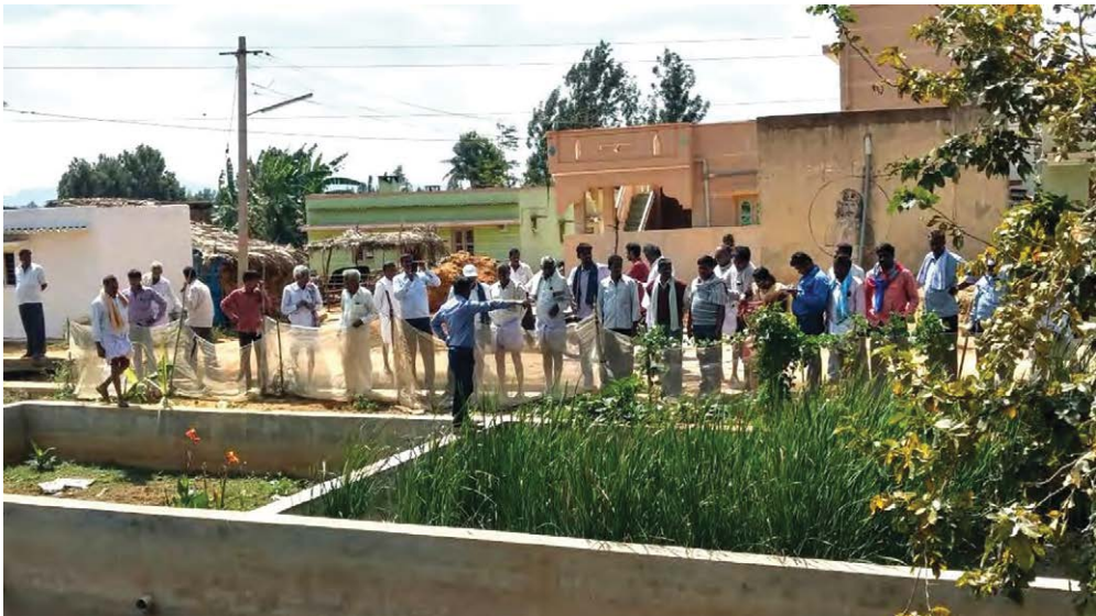
Fig. 7.15. Constructed wetland in Dandiganahalli for treating domestic wastewater.
