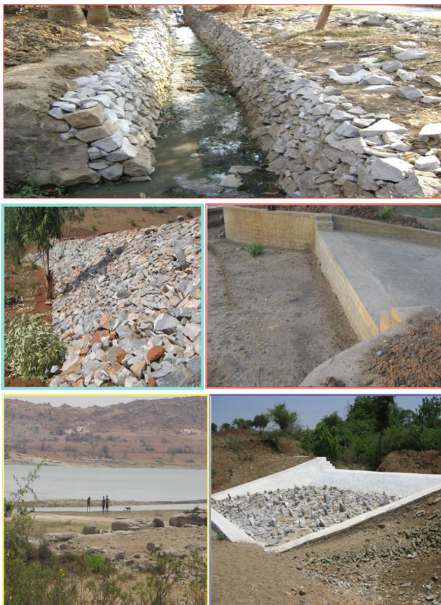
Fig. 11.4 Village development works taken up under MGNREGA
