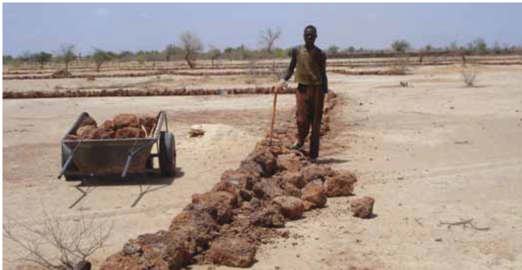
Figure 4. Implementation of the contour stone bunds. Photo: Hien F
