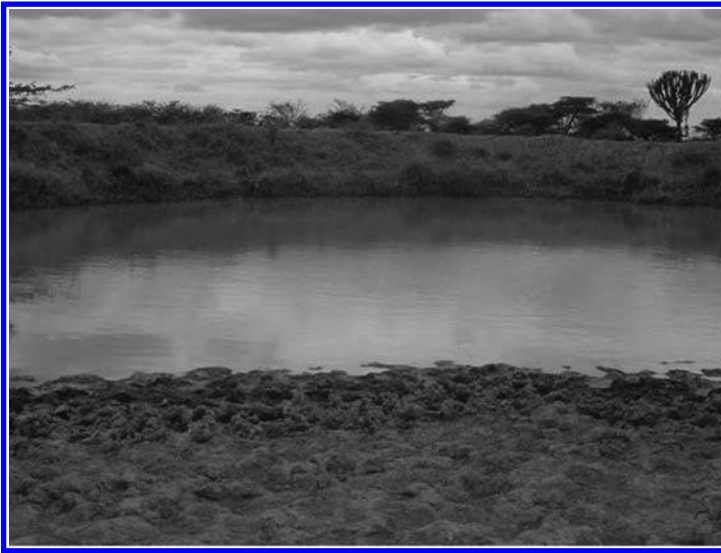
Figure 8.3 An excavated pan for holding runoff in Koibatek, Kenya
