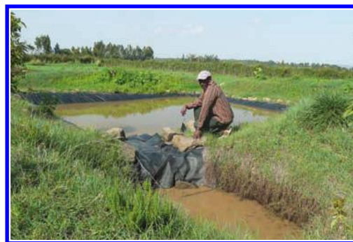
Figure 8.5 Plastic-lined pond for rainwater harvesting in Minjar Shekora, Ethiopia
